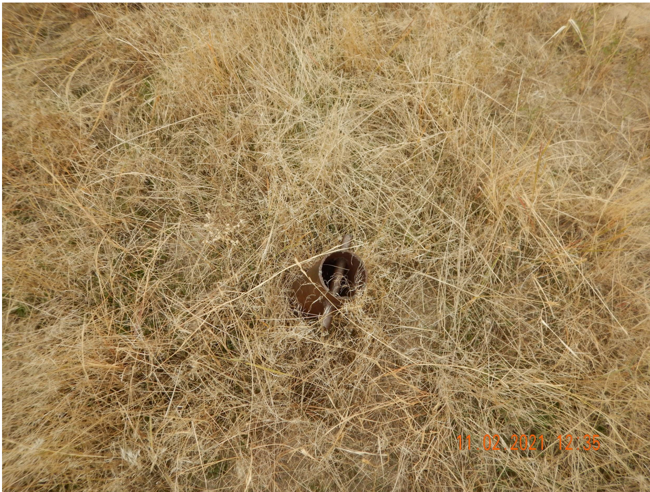
Photo 2. Photo illustrates 1 of 5 guy line anchors that have not been removed.
