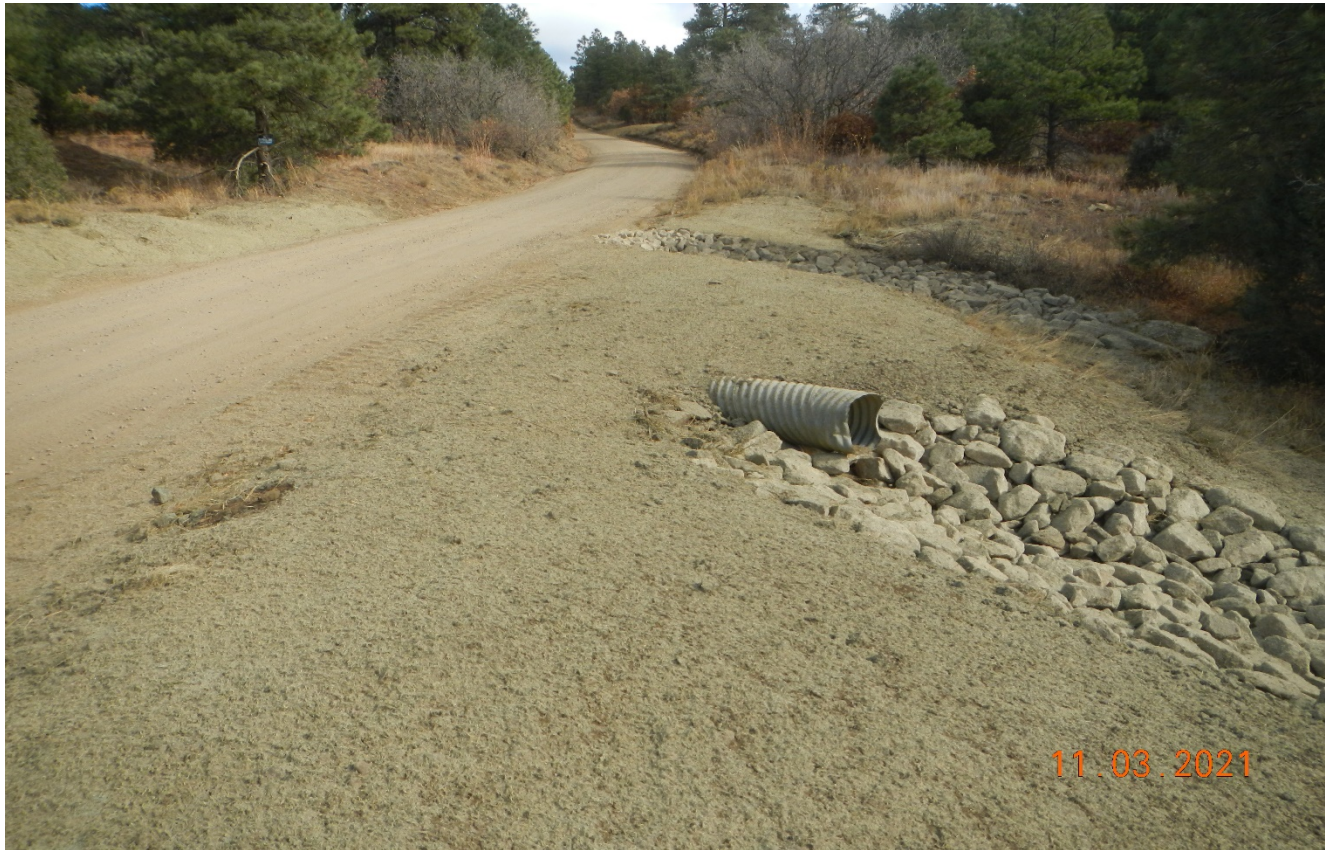
Photo 5. There are areas along the road that have been seeded and hydromulched. Outlet protection was installed at the culvert and stormwater diversion.
