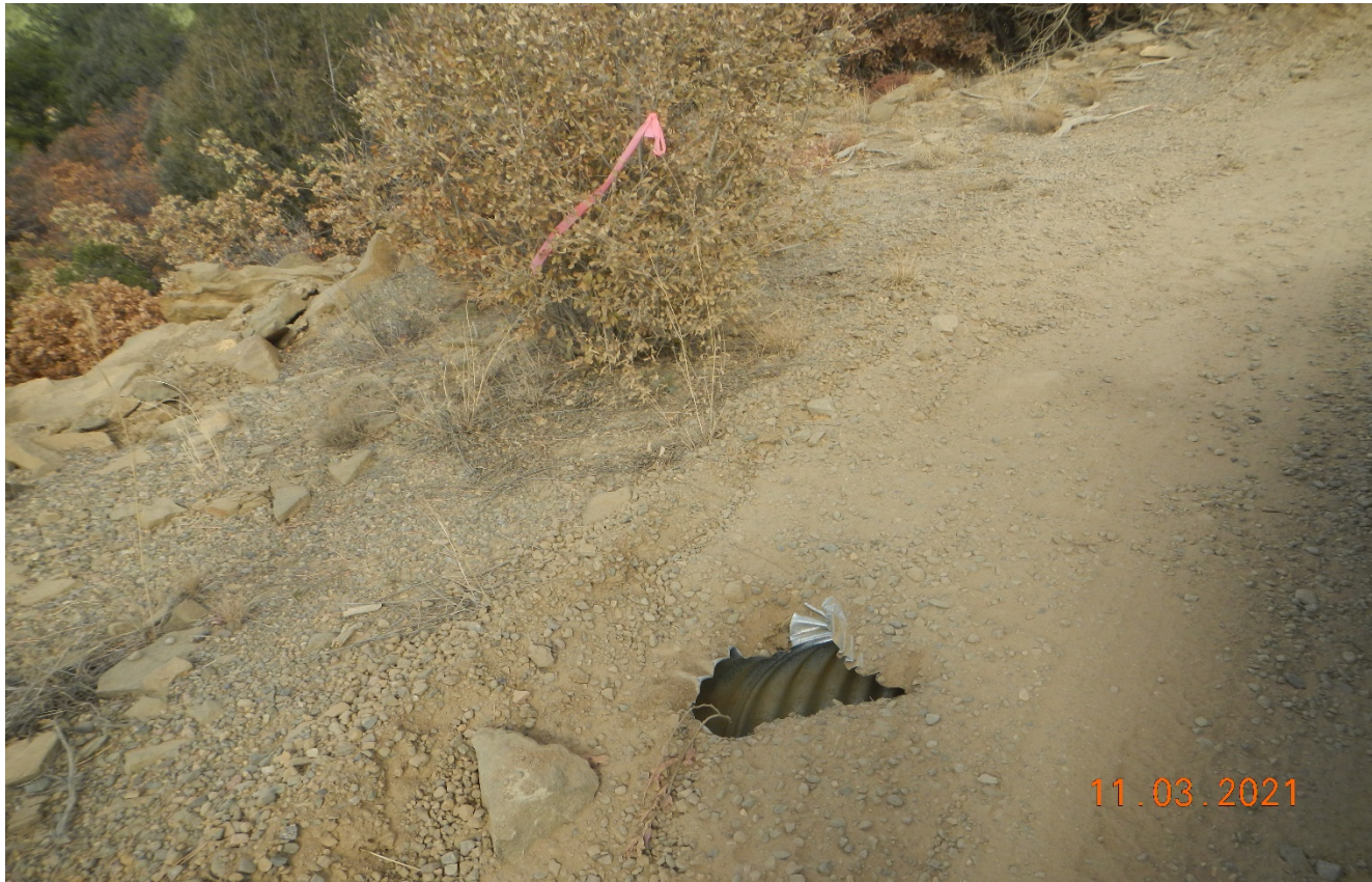
Photo 3. The culvert was damaged which can puncture a tire. This needs to be repaired. Additionally, the ribbon markers need to be removed once work is completed.
