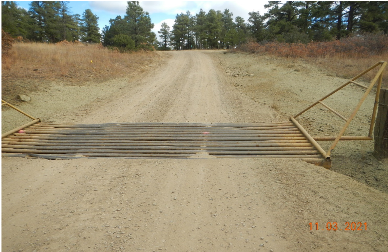
Photo 7. The cattleguard along the road has been repaired. Further up the road another cattle guard was also repaired.
