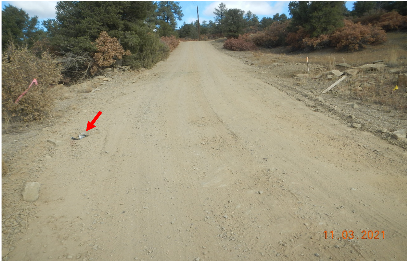
Photo 2. The access road has been regraded however there are steep areas with insufficient gravel and stabilization. The red arrow points to a culvert that was damaged from grading. Lat/Long:37.23640,-104.69944
