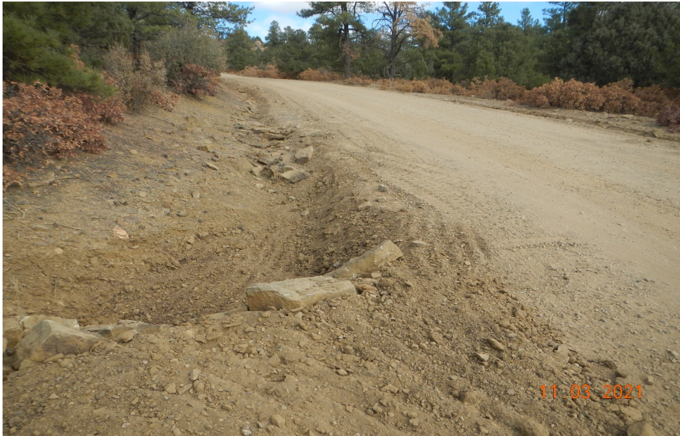
Photo 4. The culverts along the road have been cleaned out and repaired.
