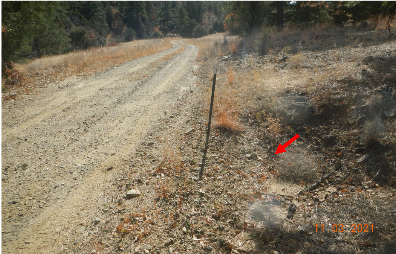
Photo 1. Facing southeast along the access road. The culvert along the road is filled in with sediment.
