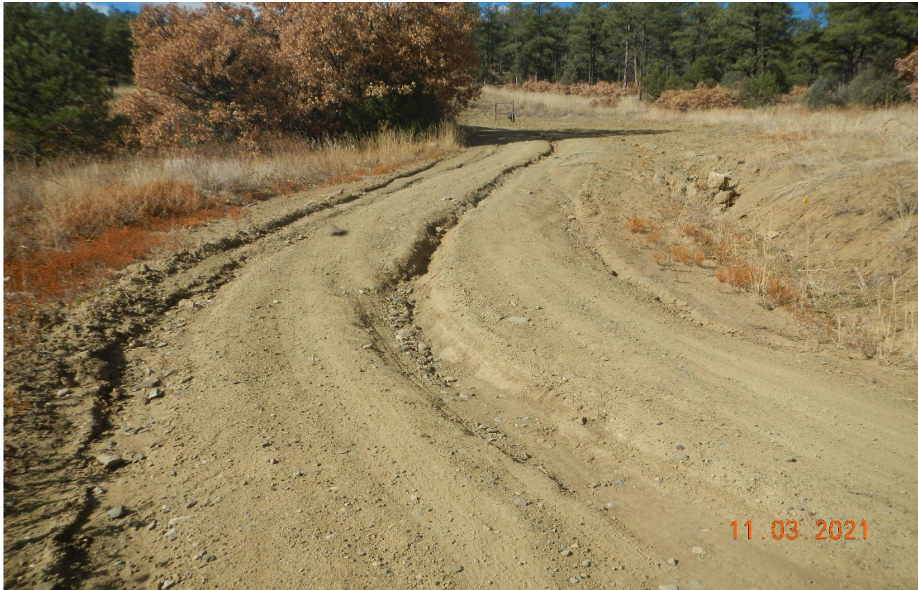
Photo 2. Facing west toward the access road near the location. There is erosion along the road which needs to be repaired and stabilized.
