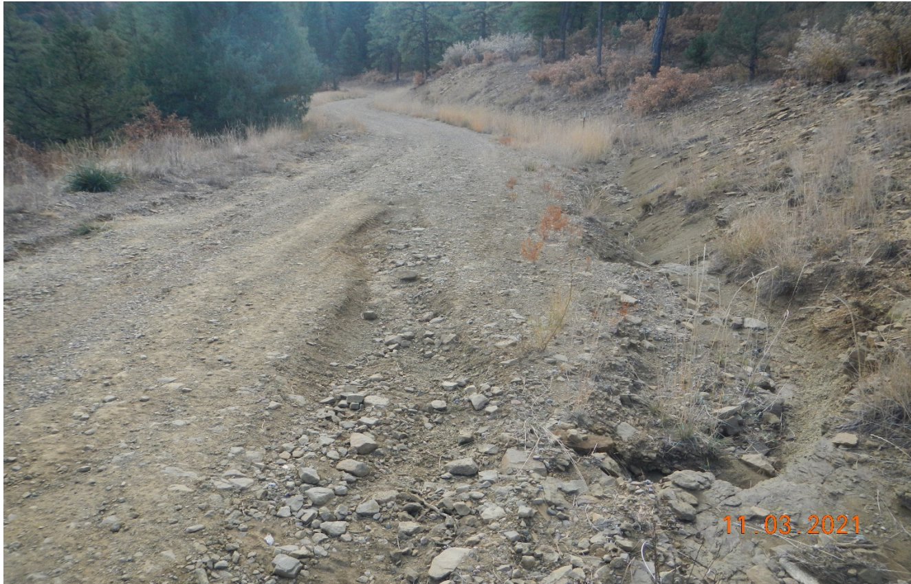
Photo 2. Facing southeast further down the road. There is erosion along the road that needs to be repaired and stabilized.
