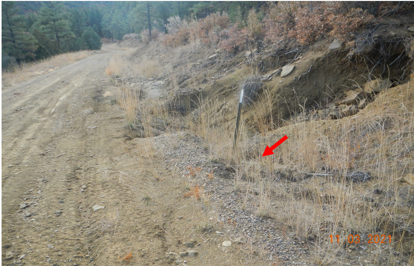
Photo 1. Facing southeast along the access road. There is an erosion gully along the road side. The culvert at red arrow is filled in with sediment and the erosion gully was measured to be 4.5 ft. deep.
