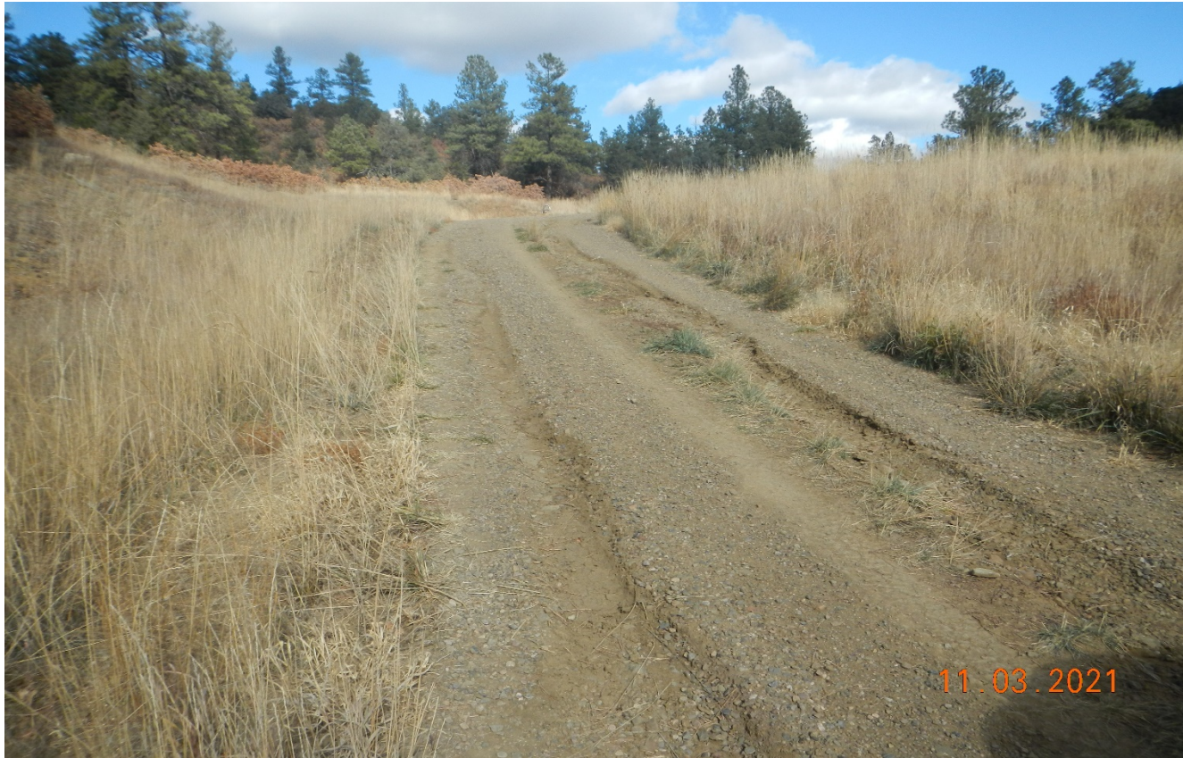
Photo 3. Facing north near the location. There is erosion along the road coming from the location.
