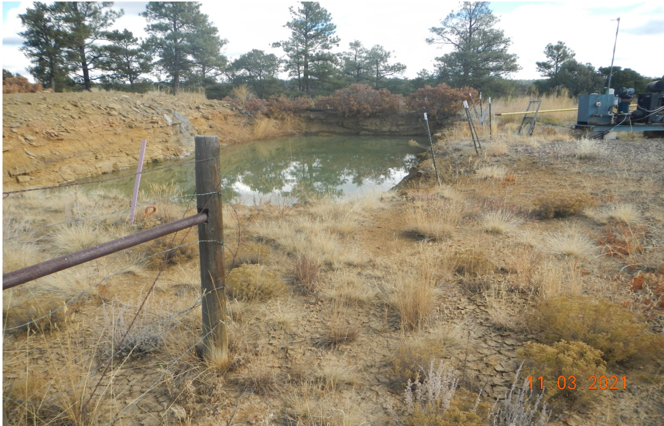
Photo 2. The fence around the pit is not maintained.
