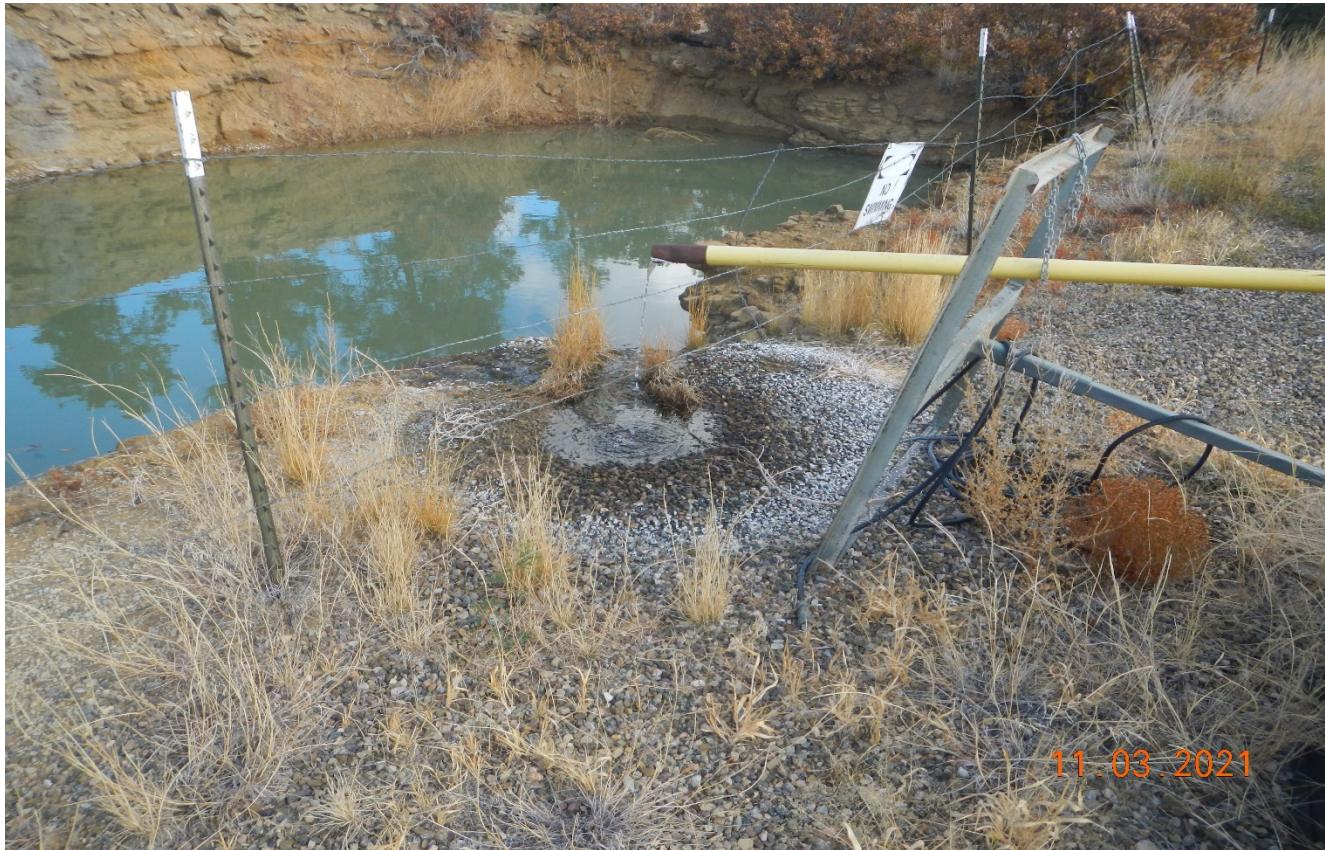
Photo 3. The PW pipe is not long enough to reach the pit.
