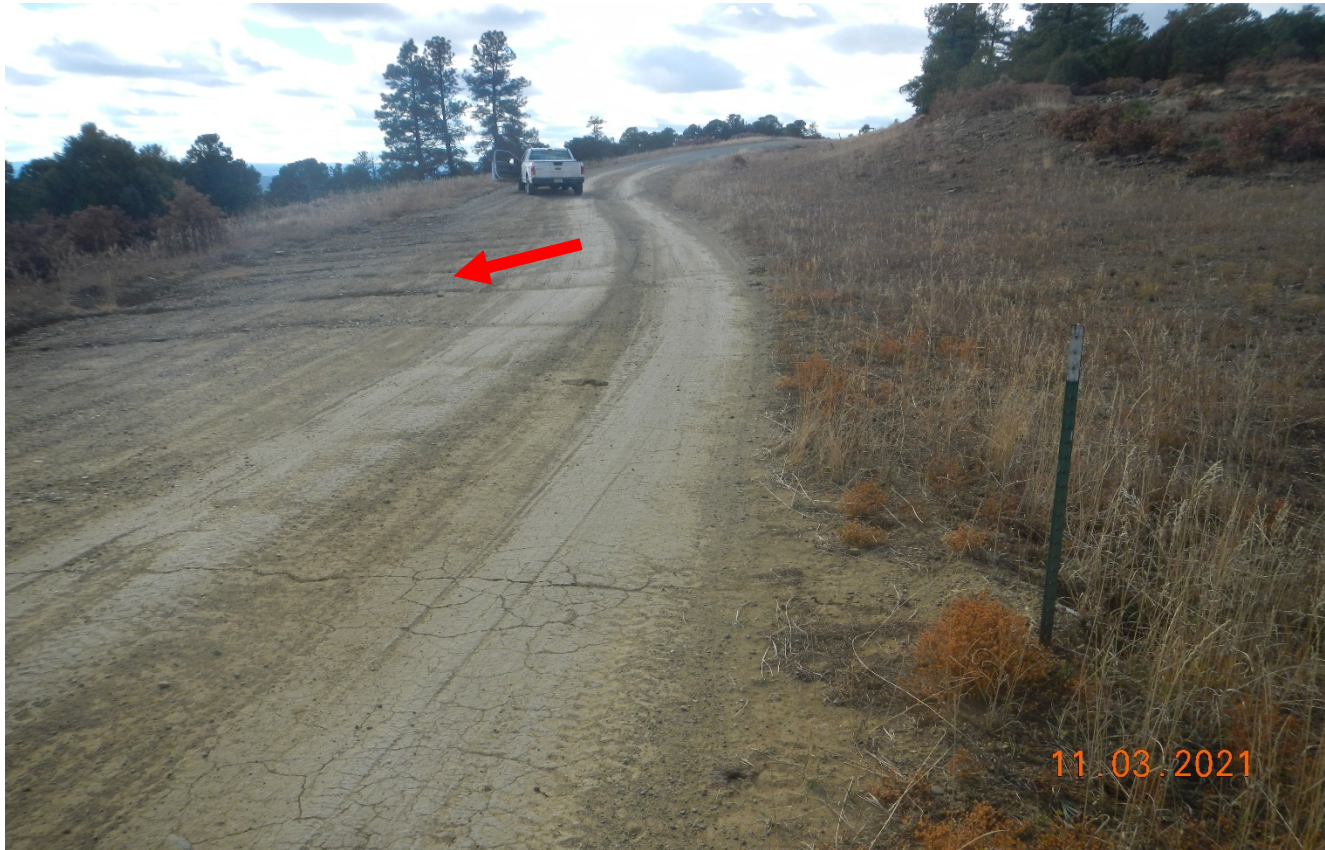
Photo 3. Facing southwest. Stormwater is flowing across the road at red arrow and is not being diverted toward the culvert.
