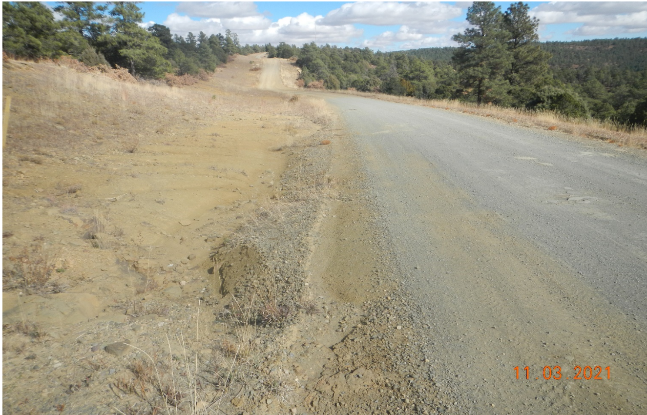
Photo 1. Facing northeast along the main access road. Stormwater erosion from this area is causing more erosion further down the road. Lat/Long:37.2354,-104.6646
