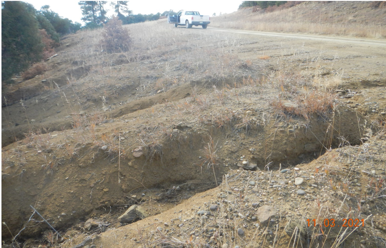
Photo 4. There is erosion along the east side of the road which needs to be repaired.
