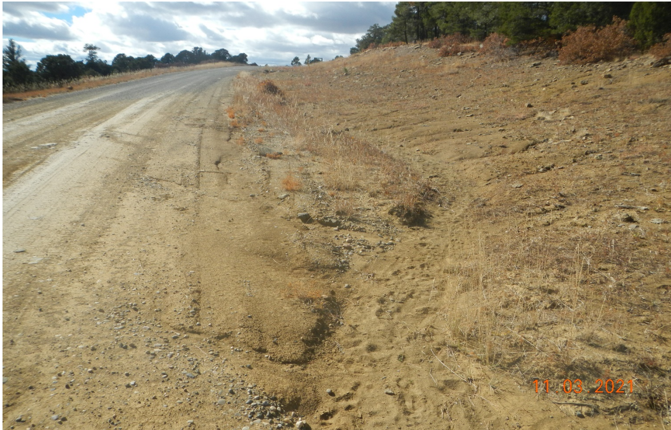
Photo 2. Facing back southwest. The road side is not stabilized and stormwater runoff is causing erosion further down the road.
