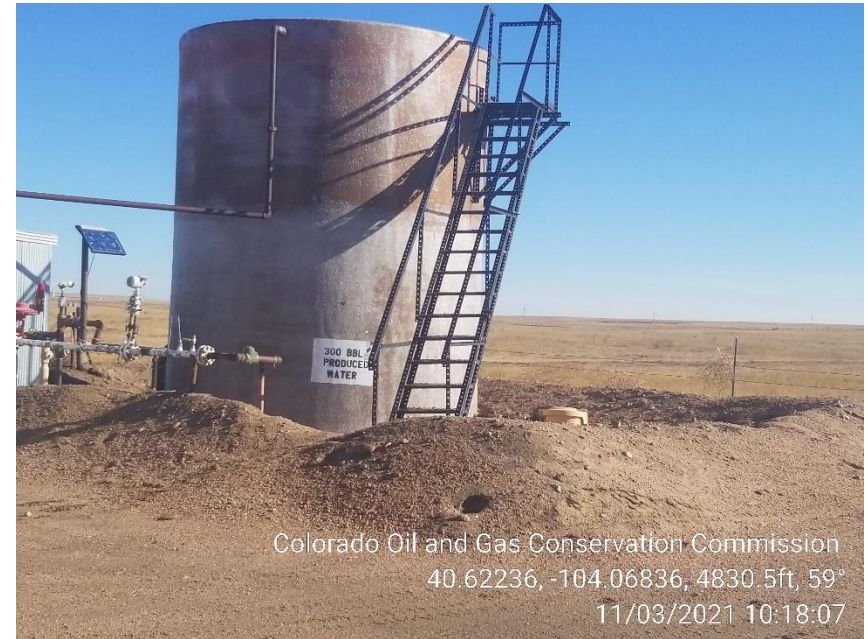
Photo 6 – Produced Water Tank
