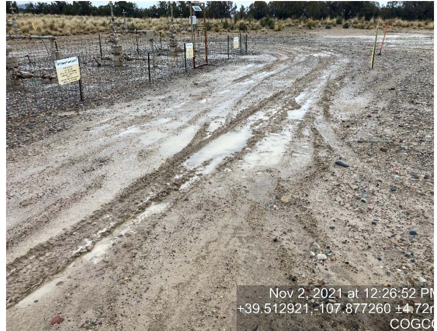
Lack of stabilization/compaction
