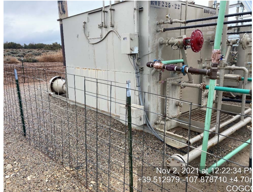
Glycol vessel lacking labeling
