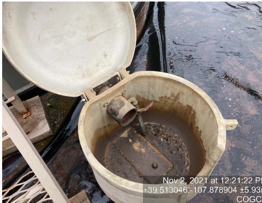
Load line missing bull plug/cap
