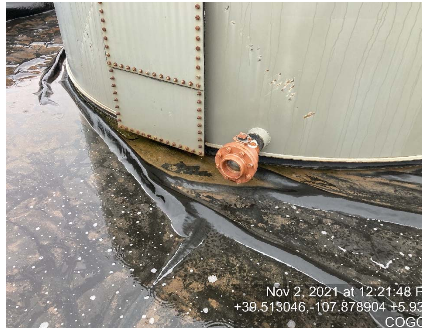
Load line missing bull plug/cap
