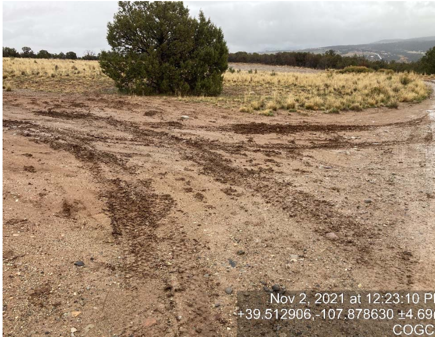
Lack of stabilization/compaction
