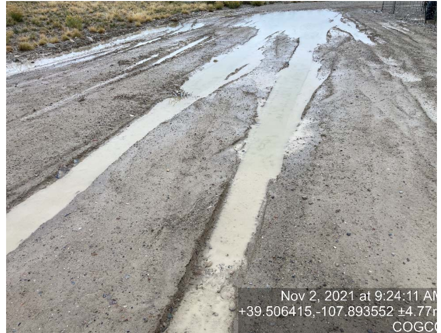
Lack of stabilization/compaction
