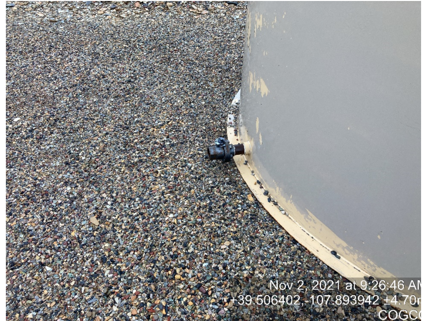
Load line missing bull plug/cap
