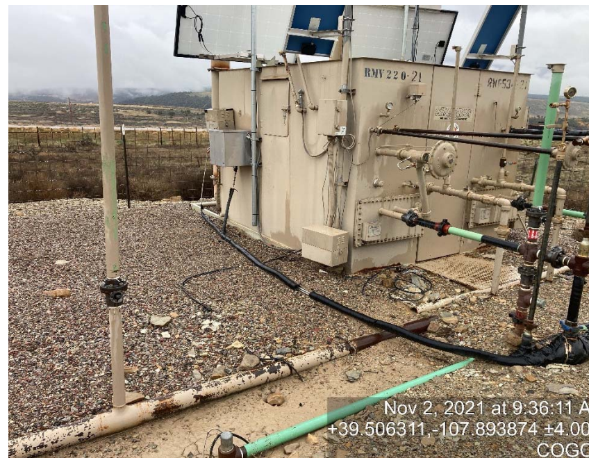
Glycol vessel missing labeling
