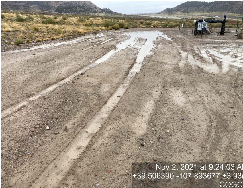
Lack of stabilization/compaction
