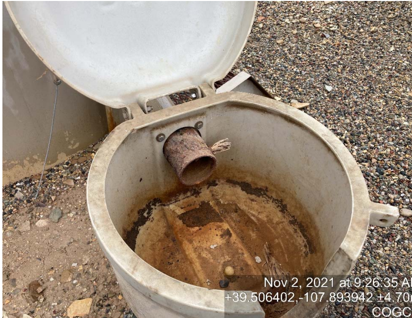
Load line missing bull plug/cap
