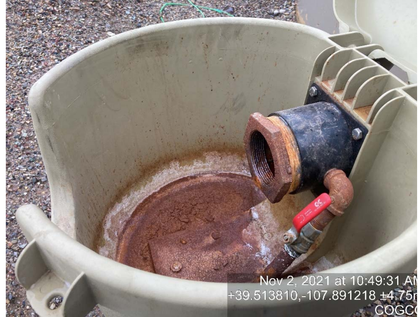
Load line missing bull plug/cap
