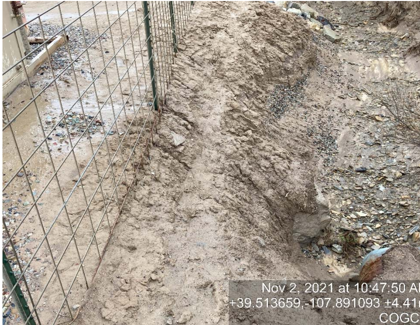
Lack of stabilization/erosion
