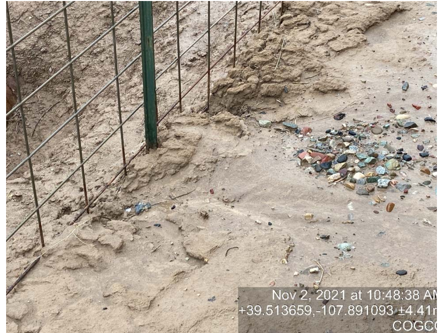
Lack of stabilization/erosion
