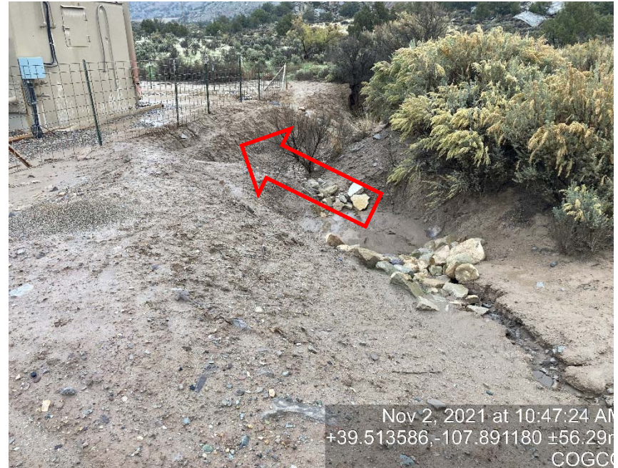
Lack of stabilization/erosion
