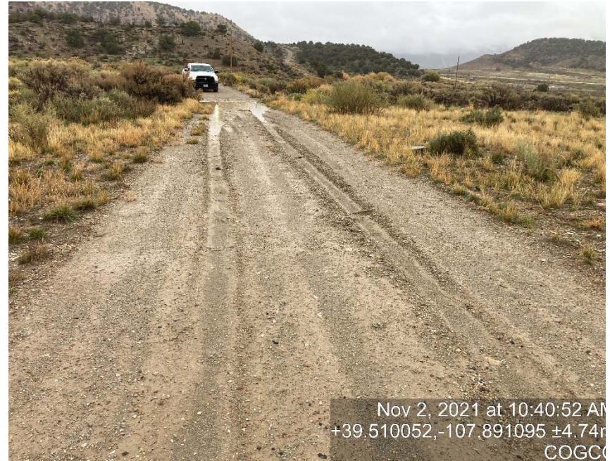
Lack of stabilization/compaction
