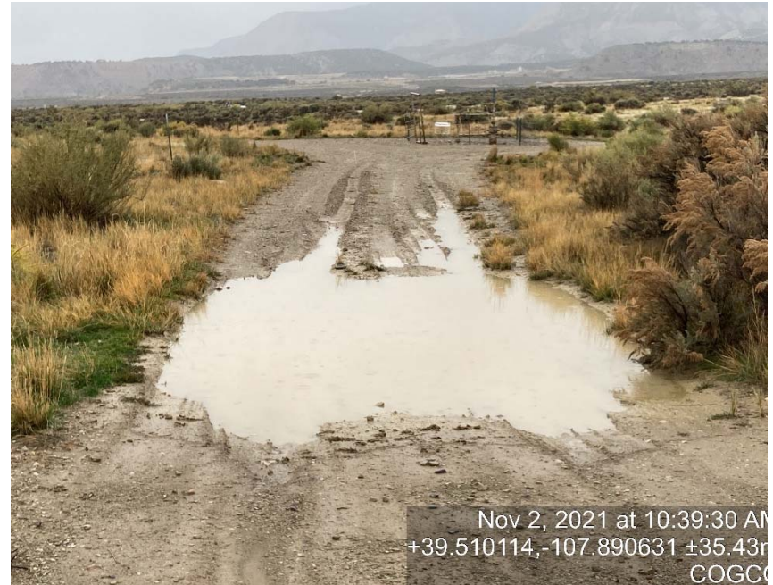
Lack of stabilization/compaction
