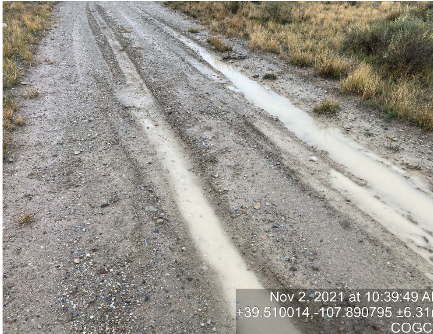
Lack of stabilization/compaction
