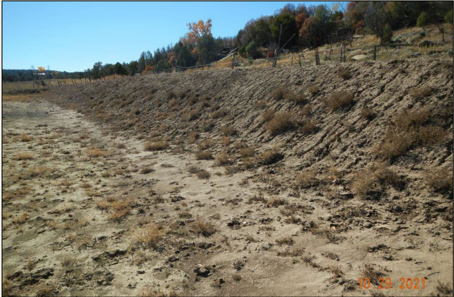
Photo 3. View of erosional rilling and sediment deposition on the well pad cut-slope. Bare soils need erosion controls until stabilized with desirable perennial vegetation.
