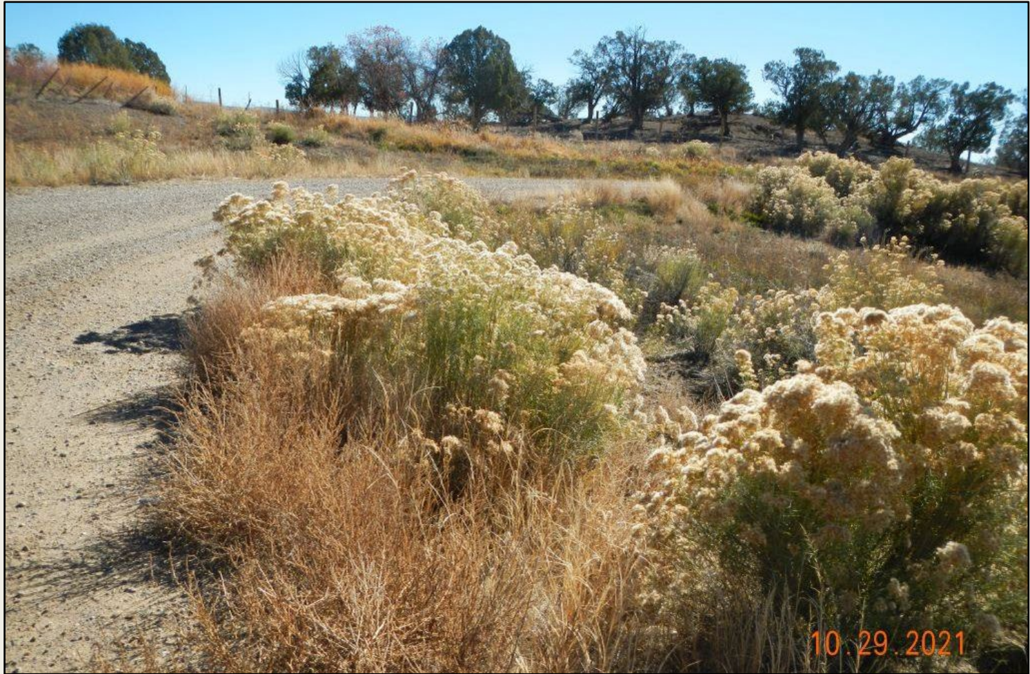
Photo 3. View of the southern fill slope from the southwestern corner facing eastward. Revegetation is progressing with rubber rabbitbrush, western wheatgrass, and sand dropseed.
