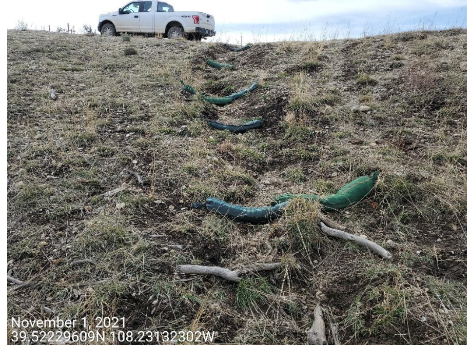
Photo 1: Photos taken from the gully erosion observed on the north end of the Location. Photos provide examples showing control measures to allow for proper stormwater discharge, and minimize erosion degradation remain missing or insufficient per good engineering practices.
