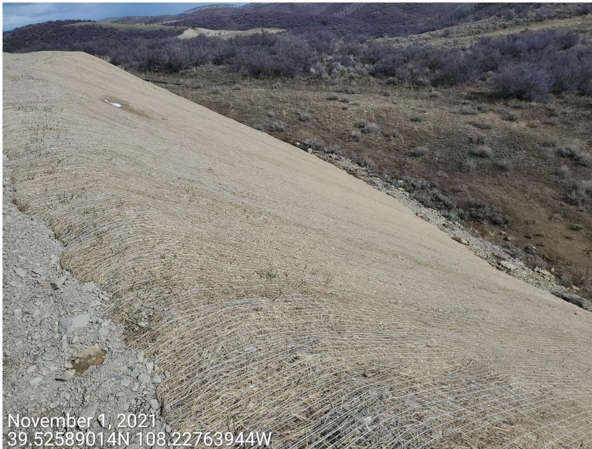
Photo 4: Photo taken from the east end of the location. Photo shows Operator has implemented erosion blankets on the bare slopes.
