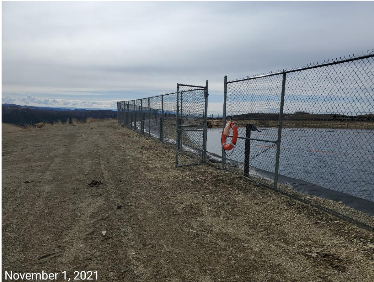
Photo 5: Photo taken from the east end of the Pond G. Photo shows gate has been left open; Best Management Practices to prevent access to the Pond G inadequate.
