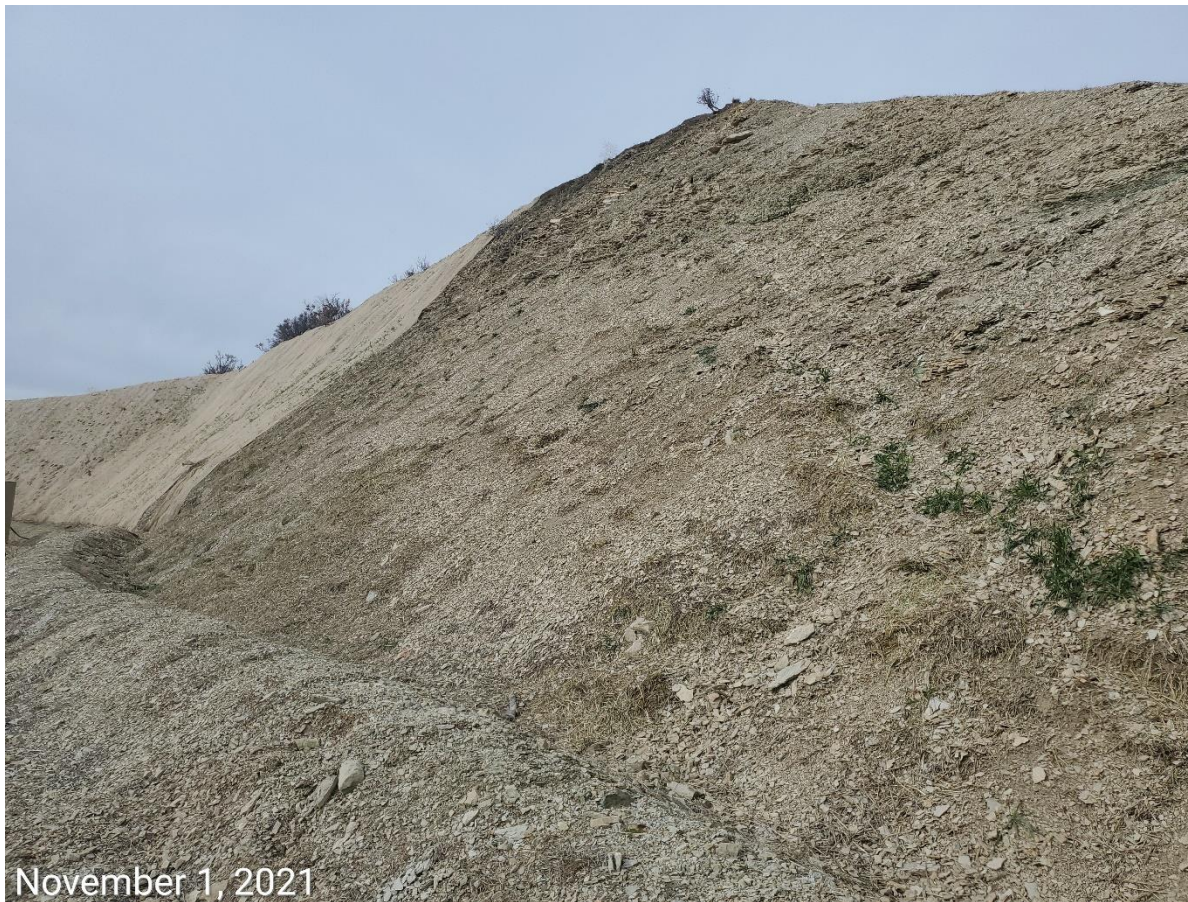
Photo 2: Photo shows large areas where control measures to protect and stabilize the cut slope remains missing or insufficient; erosion degradation evident.
