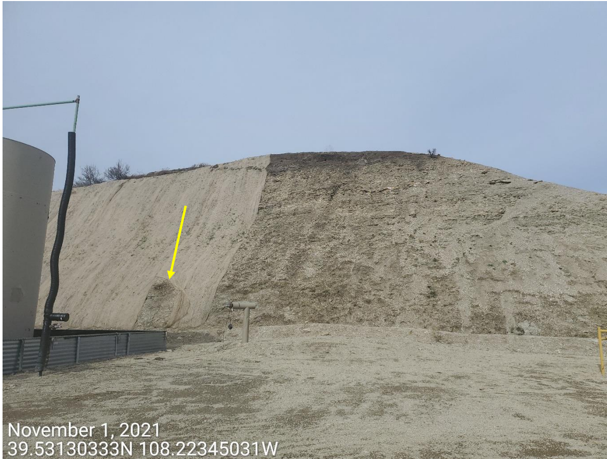
Photo 1: Photo taken from the Location, facing north. Photo shows large areas where control measures to protect and stabilize the cut slope remains missing or insufficient. Photo also shows section of erosion control blanket that has not been maintained in proper functioning condition.
