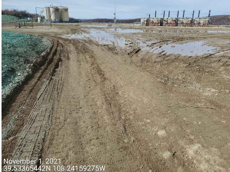
Photo 5. Photos taken from the production area and provide examples showing control measures to stabilize the Location, and mitigate tracking and offsite sediment transport are missing or insufficient.
