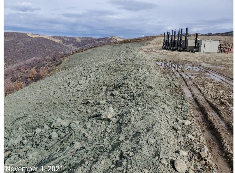
Photo 3: Photos provides example showing interim reclamation of areas not needed is in process.
