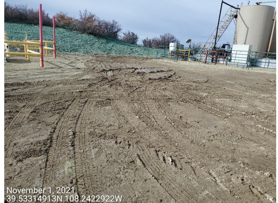
Photo 5. Photos taken from the production area and provide examples showing control measures to stabilize the Location, and mitigate tracking and offsite sediment transport are missing or insufficient.
