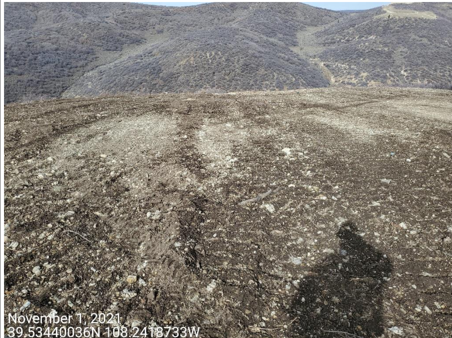
Photo 4: Photos taken from the north end of the location. Photo shows example of areas on the north end of the Location where erosion control measures to stabilize the soils are missing or insufficient.
