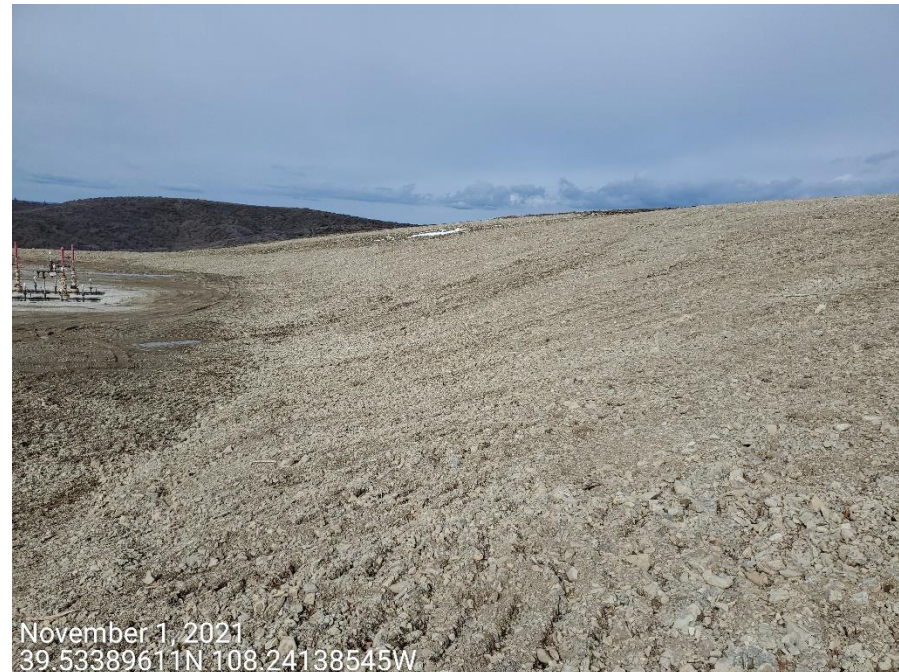
Photo 4: Photos taken from the north end of the location. Photo shows example of areas on the north end of the Location where erosion control measures to stabilize the soils are missing or insufficient.
