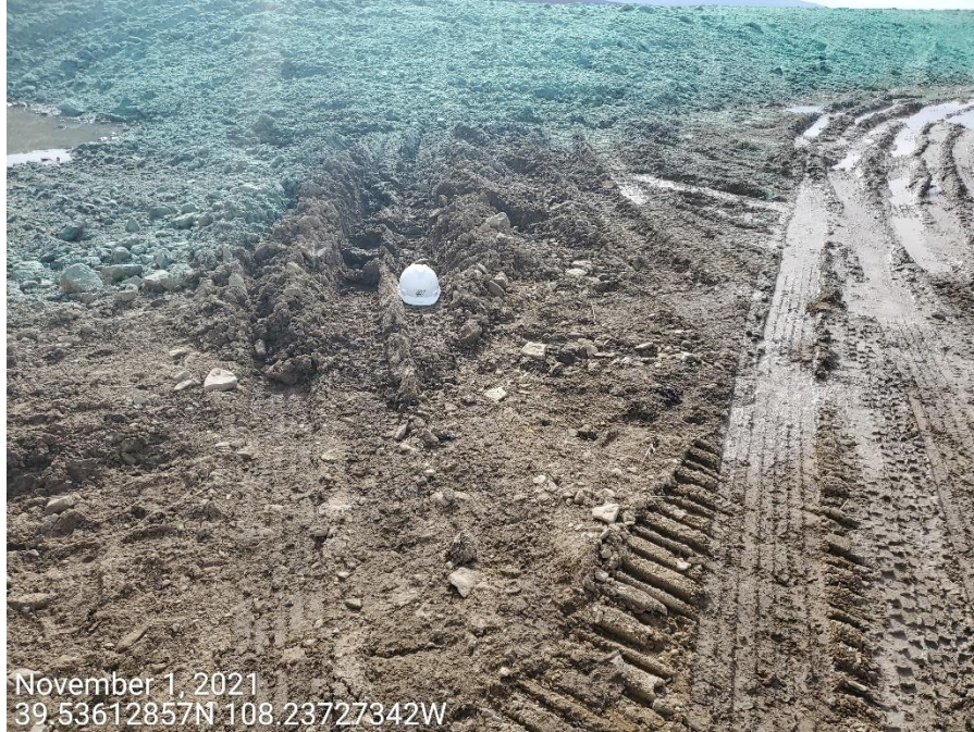
Photo 3: Photos taken from the production area and provide examples showing control measures to stabilize the Location, and mitigate tracking and offsite sediment transport are missing or insufficient.
