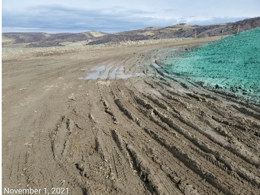
Photo 4: Photos taken from the production area and provide examples showing control measures to stabilize the Location, and mitigate tracking and offsite sediment transport are missing or insufficient. Photo on left shows Location entrance to the well pad.
