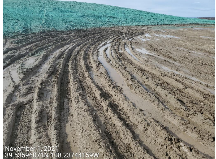
Photo 3: Photos taken from the production area and provide examples showing control measures to stabilize the Location, and mitigate tracking and offsite sediment transport are missing or insufficient.
