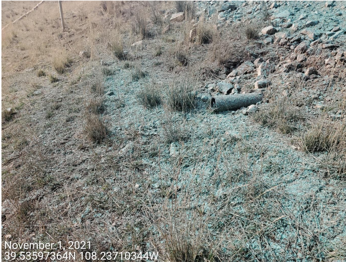
Photo 5: Photo taken from the sediment trap outlet on the east end of the Location. BMP has not been constructed in accordance with good engineering practices and is missing proper armoring and protection at the outlet spillway. Control is inadequate to allow for proper stormwater discharge.
