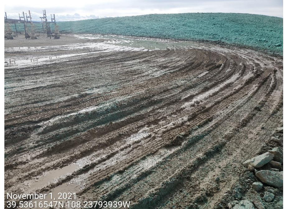
Photo 4: Photos taken from the production area and provide examples showing control measures to stabilize the Location, and mitigate tracking and offsite sediment transport are missing or insufficient. Photo on left shows Location entrance to the well pad.
