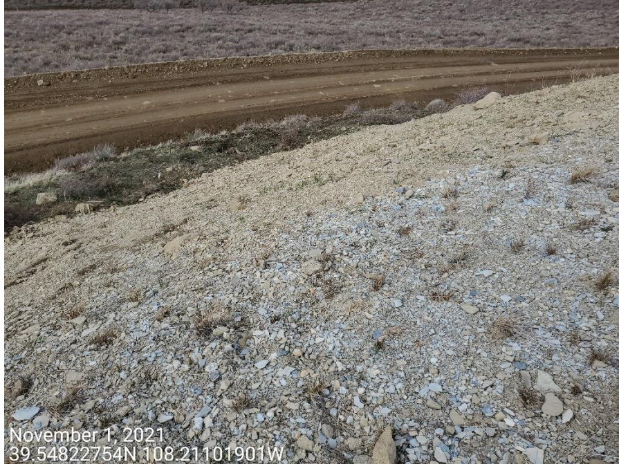
Photo 4: Photos provide examples of the slopes of the Location. Stormwater and erosion control measures to stabilize and protect the slopes, and to allow for sediment laden-free stormwater discharge remain missing or insufficient.
