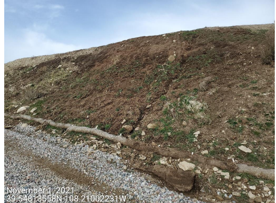
Photo 4: Photos provide examples of the slopes of the Location. Stormwater and erosion control measures to stabilize and protect the slopes, and to allow for sediment laden-free stormwater discharge remain missing or insufficient.
