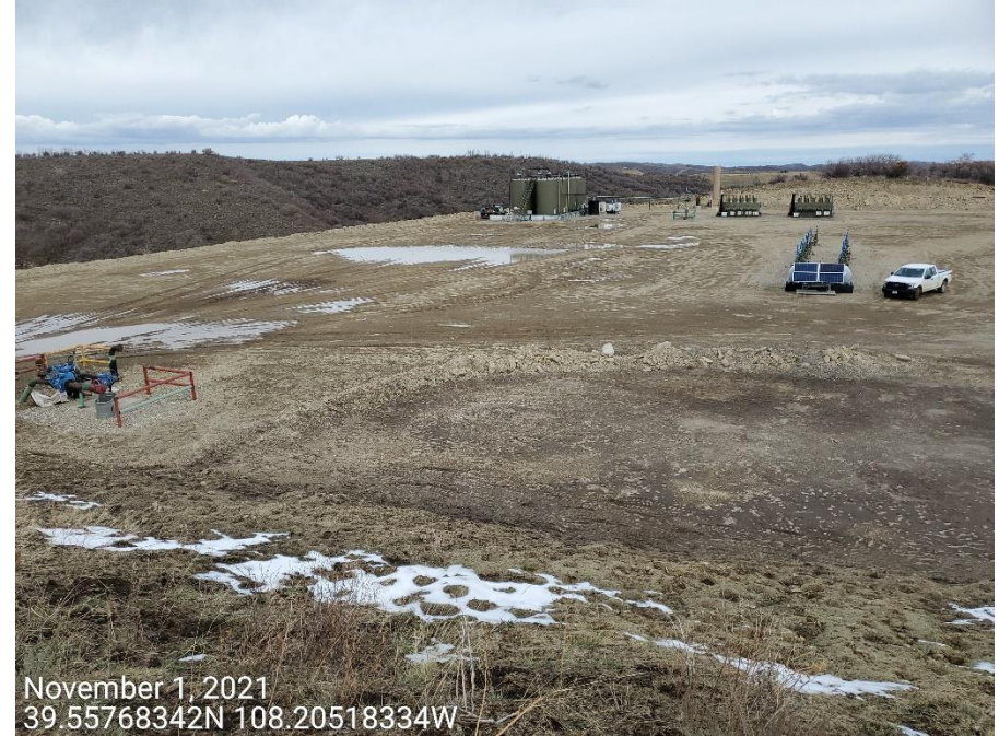
Photo 1: Photos 1-2 taken from the south end of the Location. Photos provide an overview of the Location from west, northwest, northeast to east. Photos also show interim reclamation has not been conducted on the location in accordance with 1003 rules.
