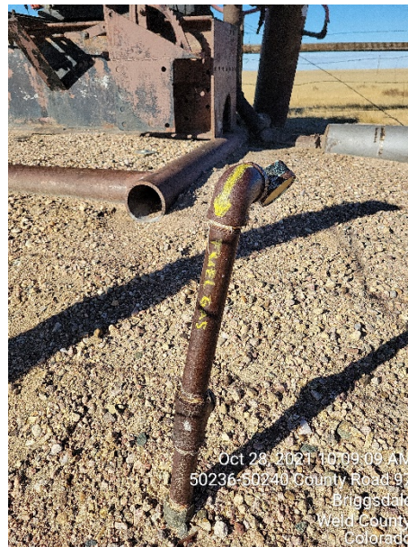
Photo 3 – Unmarked 1” Riser – Marked ‘Fuel Gas’
