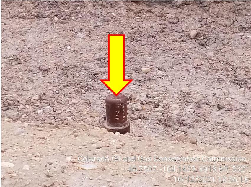
**Photo 3 – Marking is fading**
