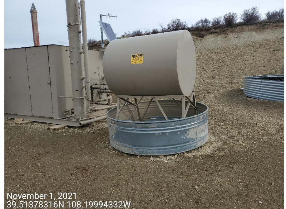
Photo 1: Photo show wildlife protection devices to prevent wildlife access to the secondary containment BMPs are missing.
