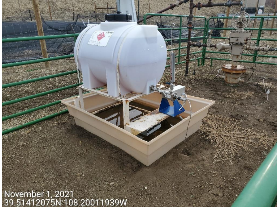
Photo 1: Photo show wildlife protection devices to prevent wildlife access to the secondary containment BMPs are missing.
