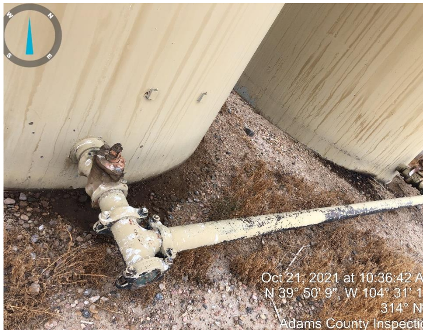
Photo #4 Stained soil on the back side of crude tanks
