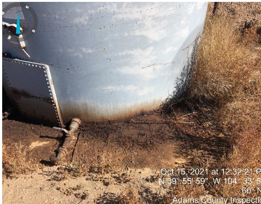
Photo #4 Stained soil around tank
