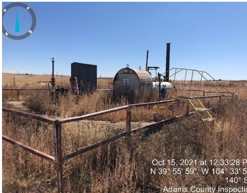
Photo #2 Meter run & Separator.
