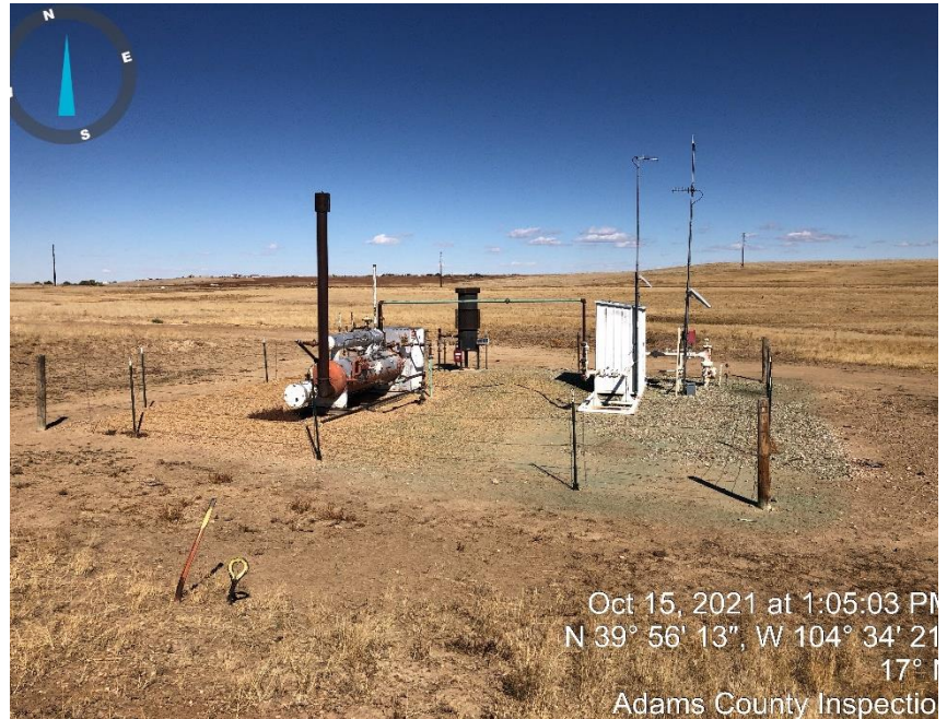
Photo #2 Separator, ECD & Meter run.
