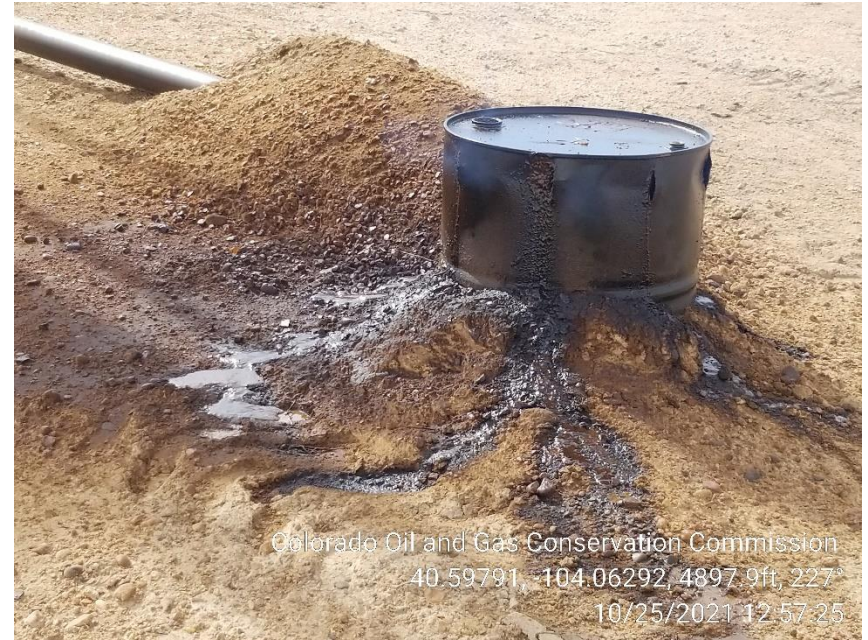
Photo 12 – Stained Soil at 2-1H Exhaust
