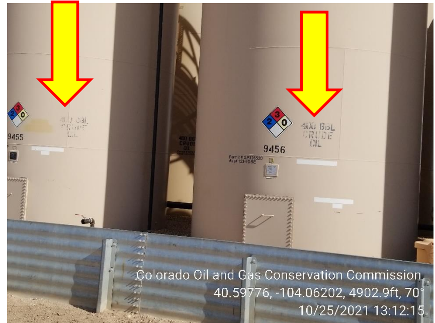
Photo 16 – Content and Capacity faded
