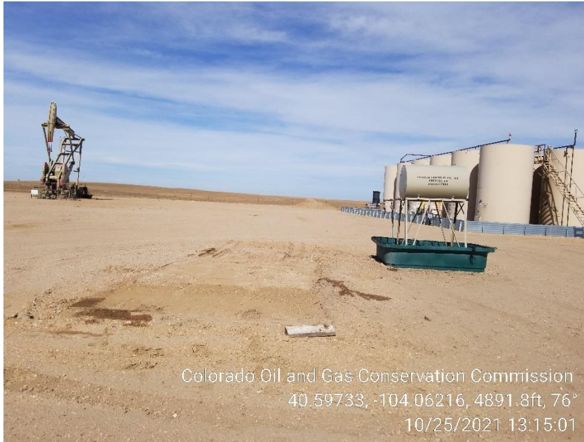
Photo 19 – Stained Soil where Compressor was located
