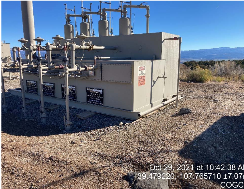
Location/lack of glycol vessel labeling
