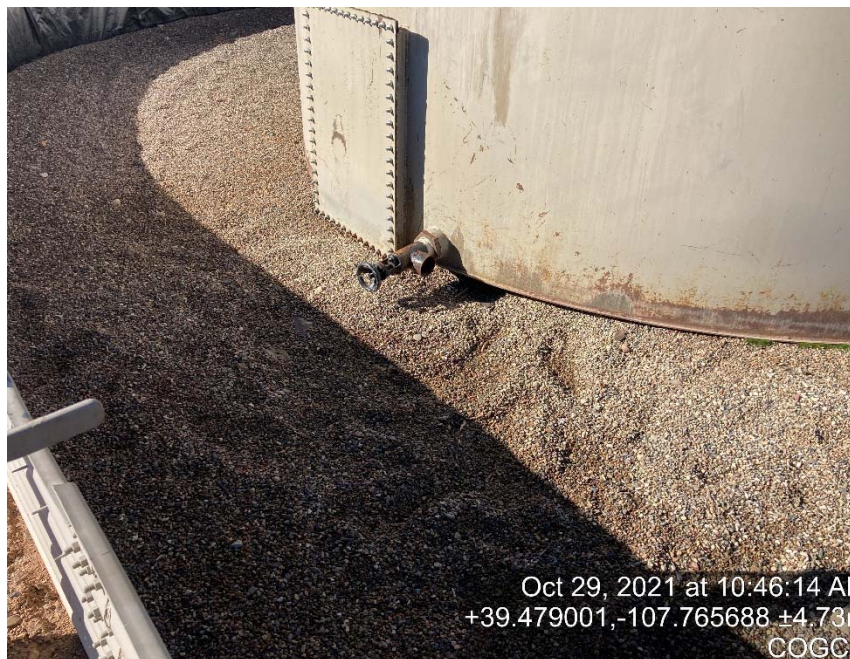
Missing load out cap/bull plug
