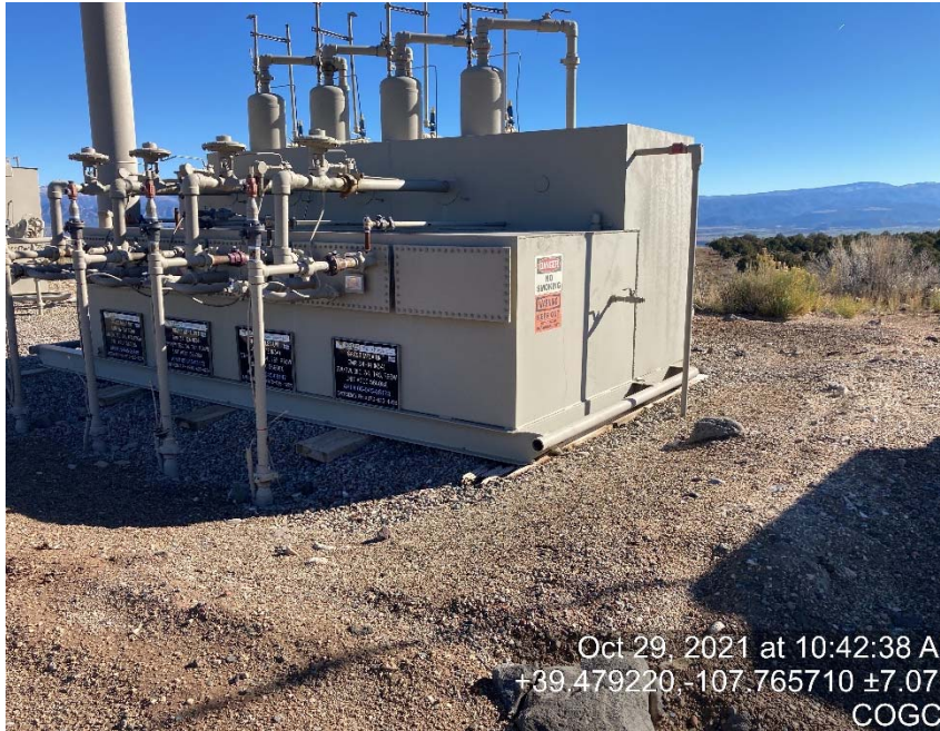
Location/lack of glycol vessel labeling
