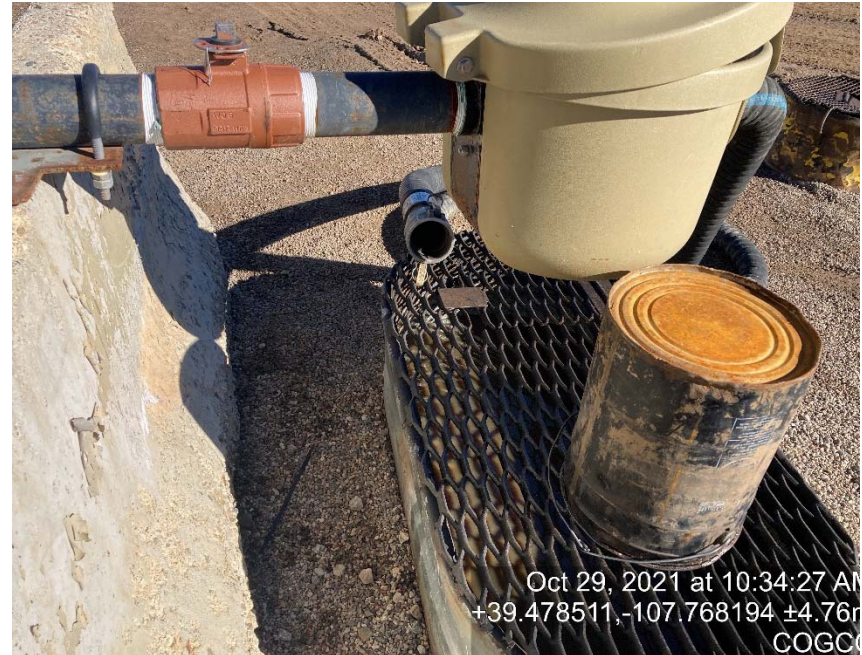
Load line missing cap
