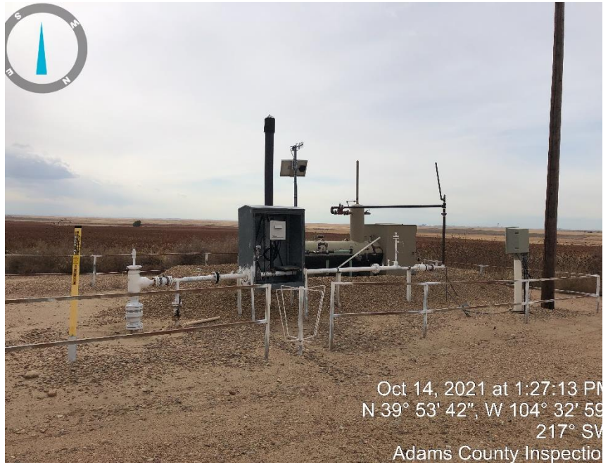
Photo #2 Meter run & Separator.
