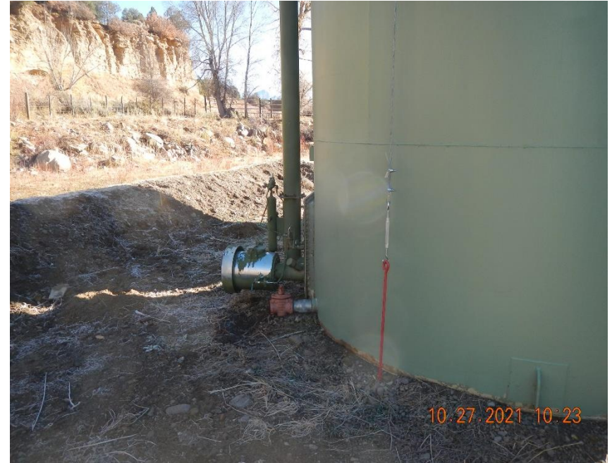
ASTs have been attached to anchors.
