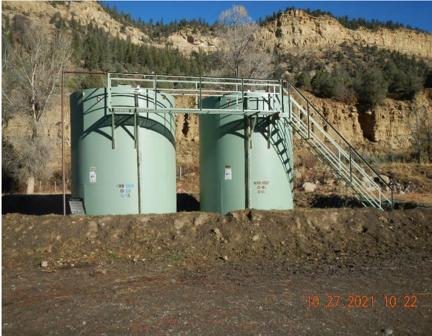
Albert Martinez #1 tank battery. Uncompacted earthen berm shared with Nielson #4 AST.
