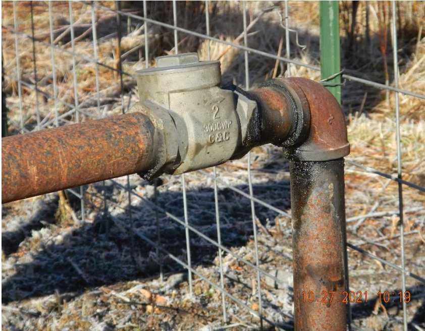
Oil staining near flow line elbow.
