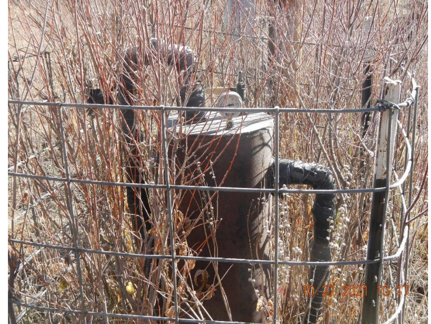
Domestic tap #477321. Pressure gauge reads approximately 14 psi.
