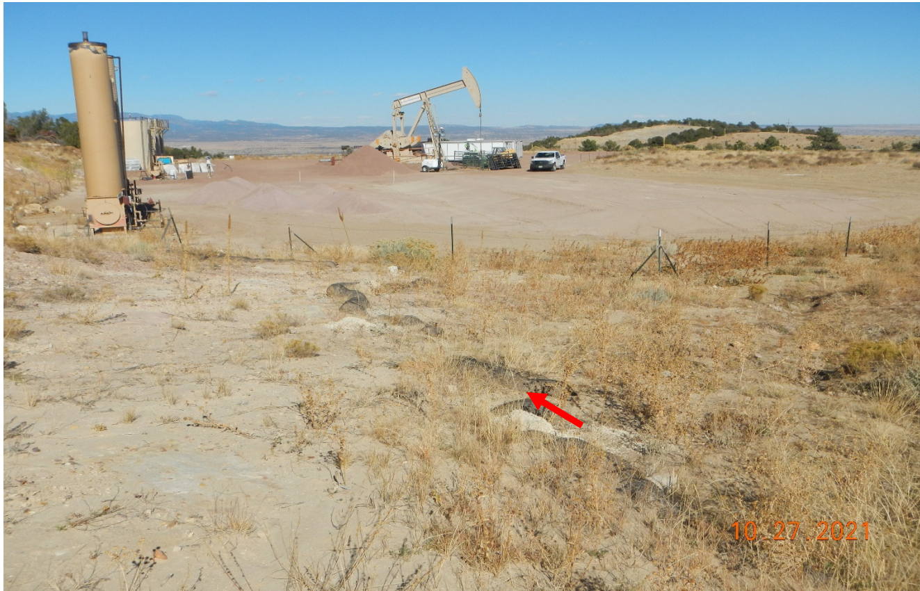
Photo 7. Facing northwest toward the location. The degraded wattles remain in this area and erosion has not been repaired.
