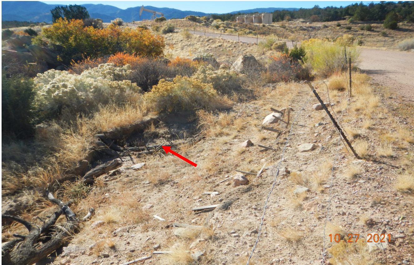
Photo 1. Facing southwest along the access road. Stormwater from the road is creating erosion in area shown at red arrow. The wattles placed in this area are displaced and are not controlling erosion. Previous corrective action has not been performed.
