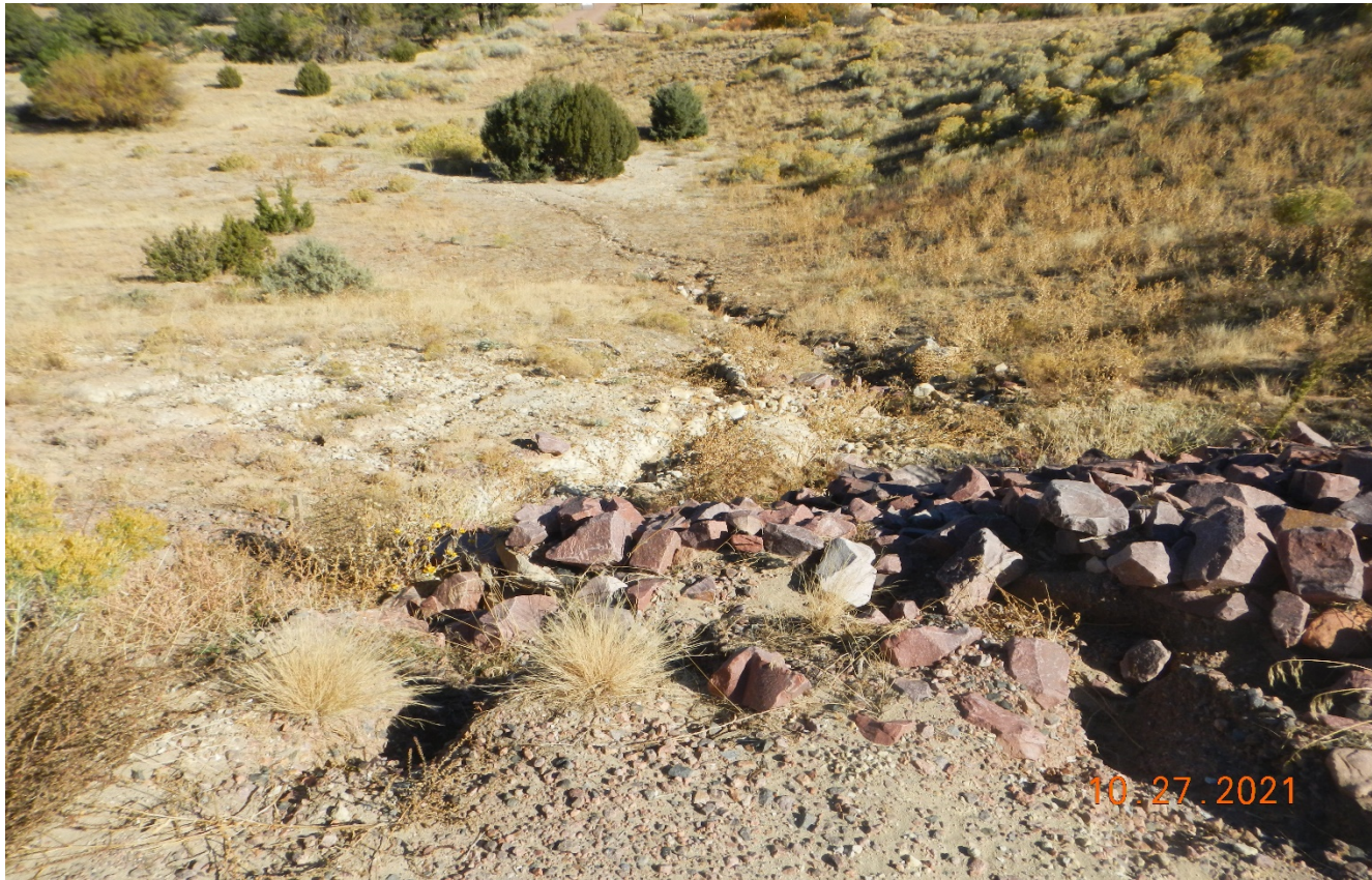
Photo 14. There is erosion occurring across the road at the north side of the location caused by stormwater directed from the top perimeter ditch shown in the previous photo. Previous corrective action has not been performed.
