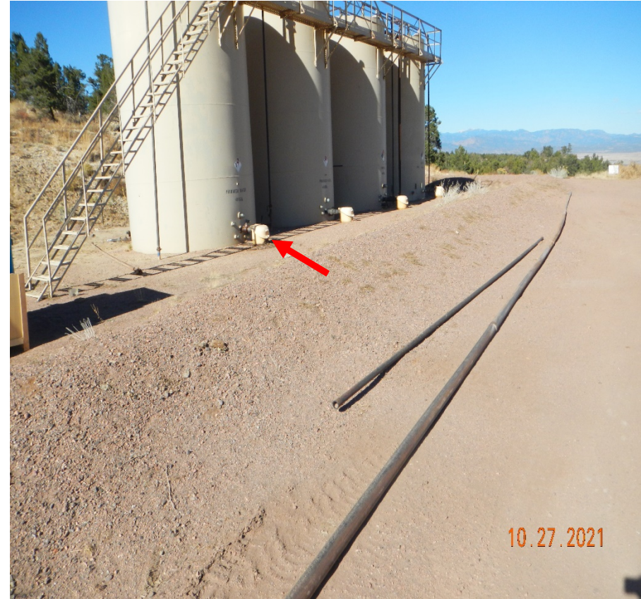
Photo 12. There is stained soil at the outlet of the PW tank which has not been cleaned up. There is also unused pipe storage at the base of the berm.
