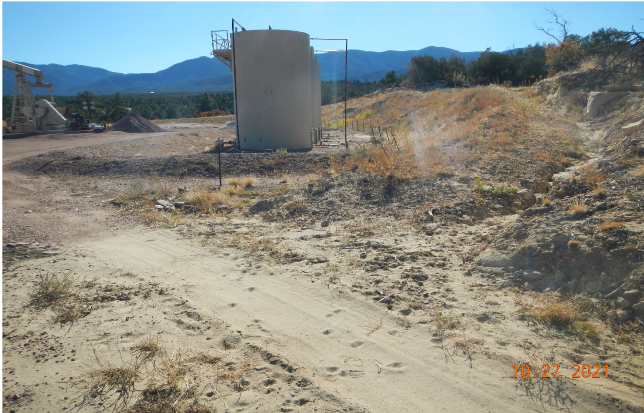
Photo 13. The top perimeter ditch is directing stormwater toward the road which has deposited sediment onto the road. BMP's are needed in this area. Previous corrective action has not been performed.
