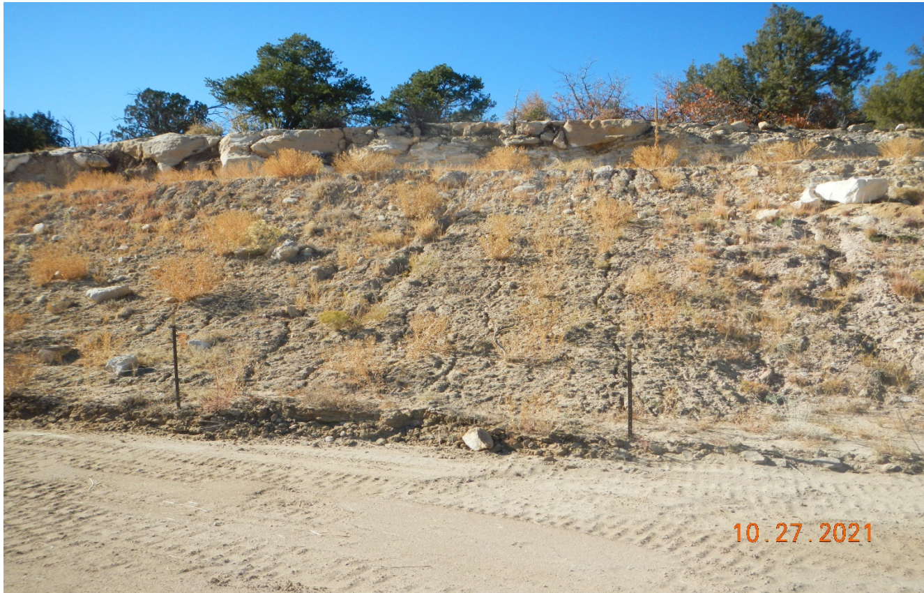
Photo 9. There is erosion along the cut slope which has not been repaired.
