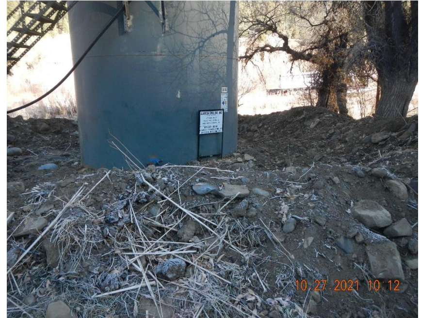
Uncompacted earthen berm does not appear to be sufficiently impervious to adequately contain releases.
