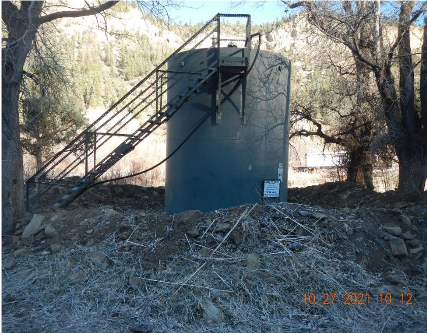
Uncompacted earthen berm around AST.
