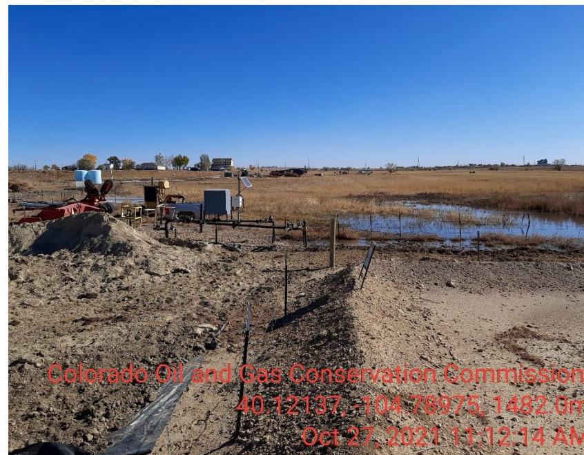
Photo 18 No BMP's around contaminated soil pile
