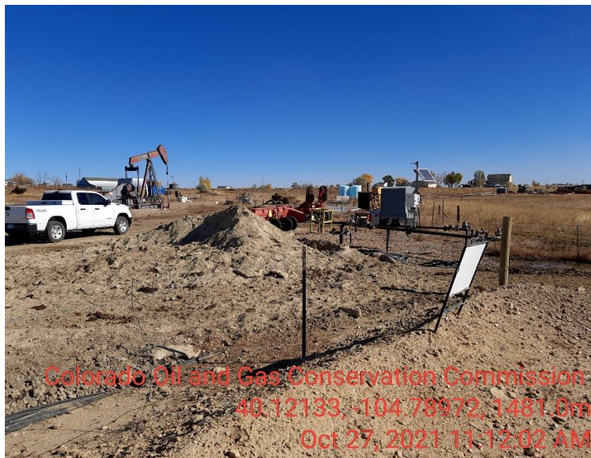
Photo 17 No BMP's around contaminated soil pile
