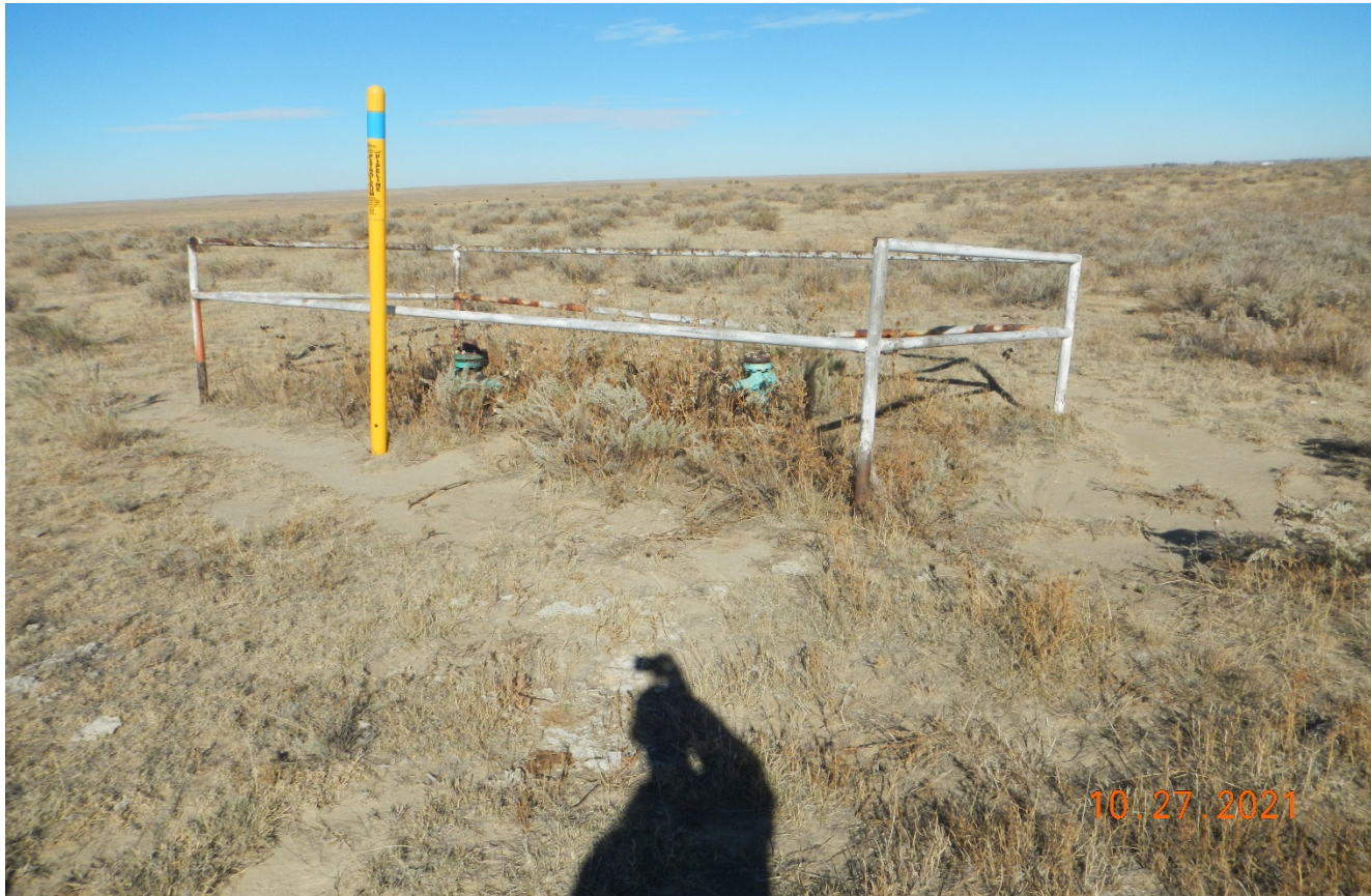
Photo 7. There are additional abandoned risers that remain at the tank battery site. All abandoned risers need to be removed.
