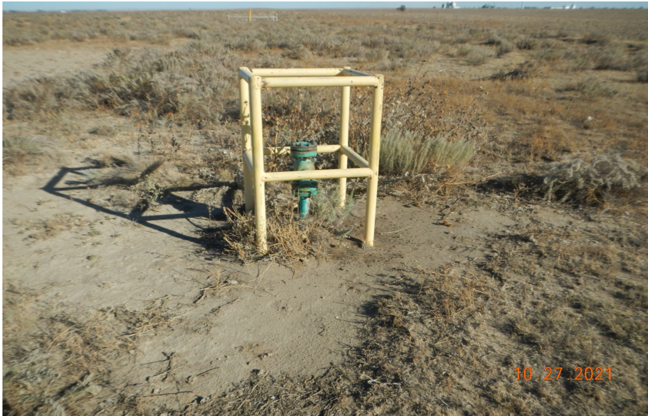
Photo 4. There is a pipe riser that remains at the battery site. All abandoned risers need to be removed.
