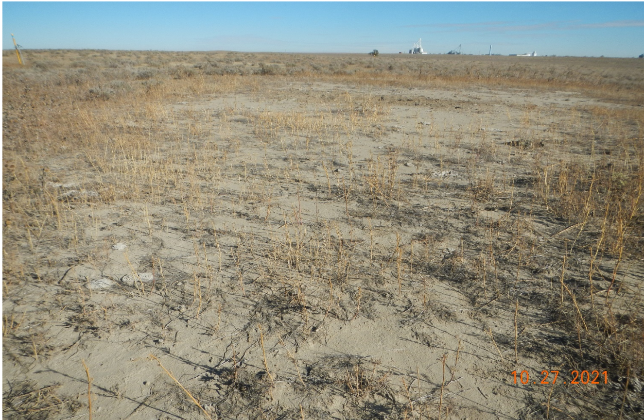
Photo 8. Facing northeast toward the abandoned well site. This area has not been reclaimed. Bare soils that are not stabilized and are susceptible to further erosion.
