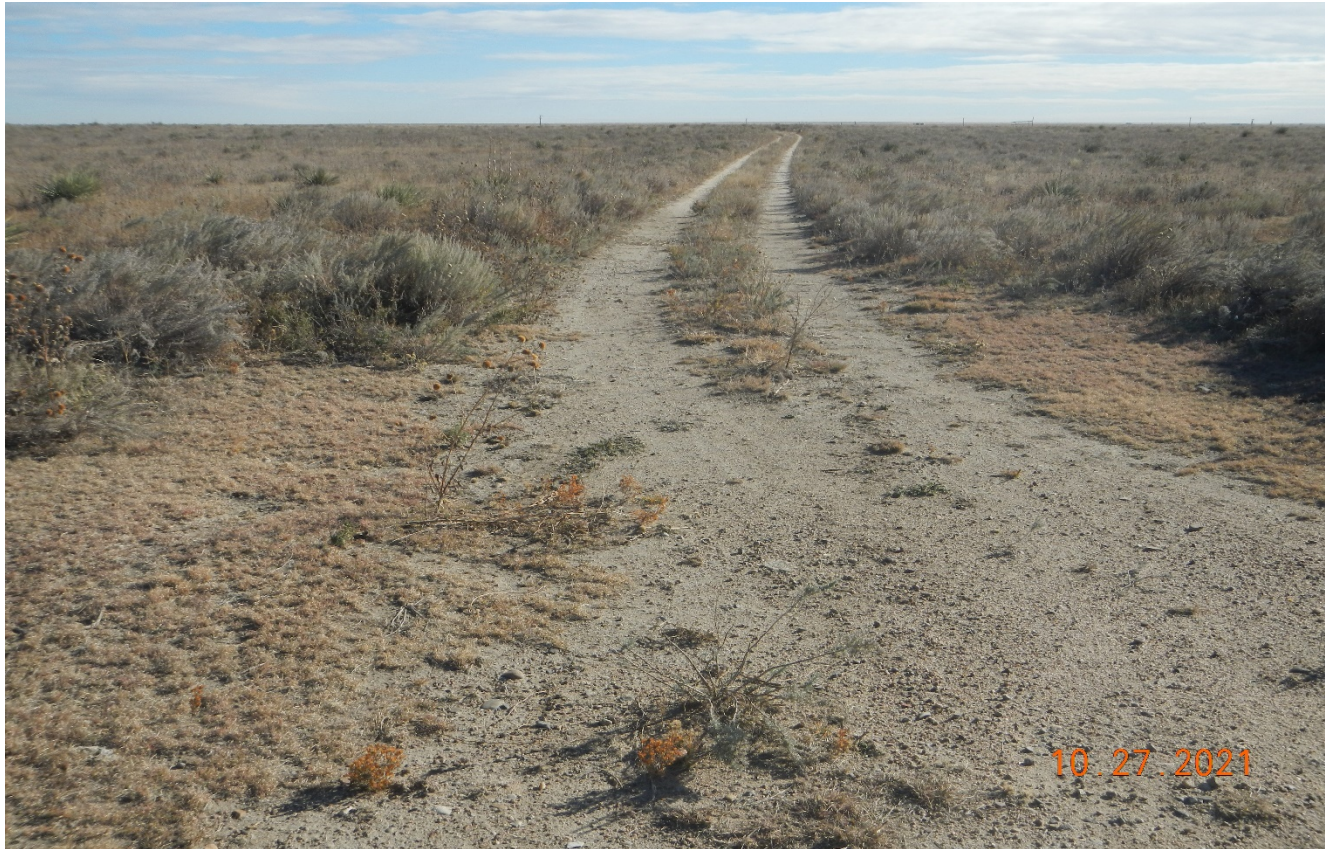
Photo 1. Facing east at the beginning of the access road. The two track road remains with compacted soils. The access road needs to be recontoured and reclaimed.
