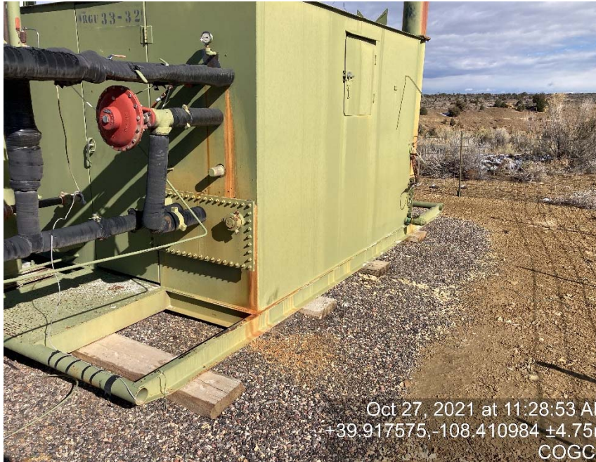
Location/lack of glycol vessel labeling
