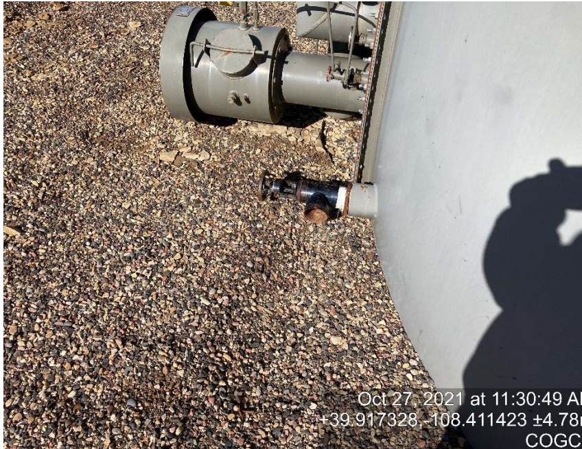
Load out line missing cap/bull plug
