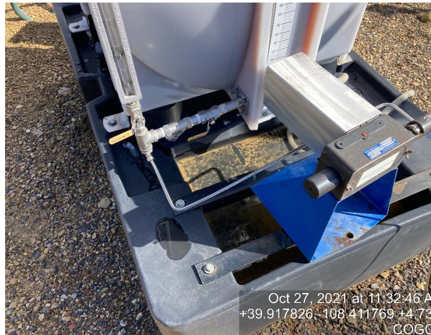
Chemical containment is full of fluid
