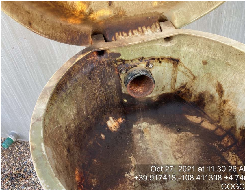
Load out line missing cap/bull plug
