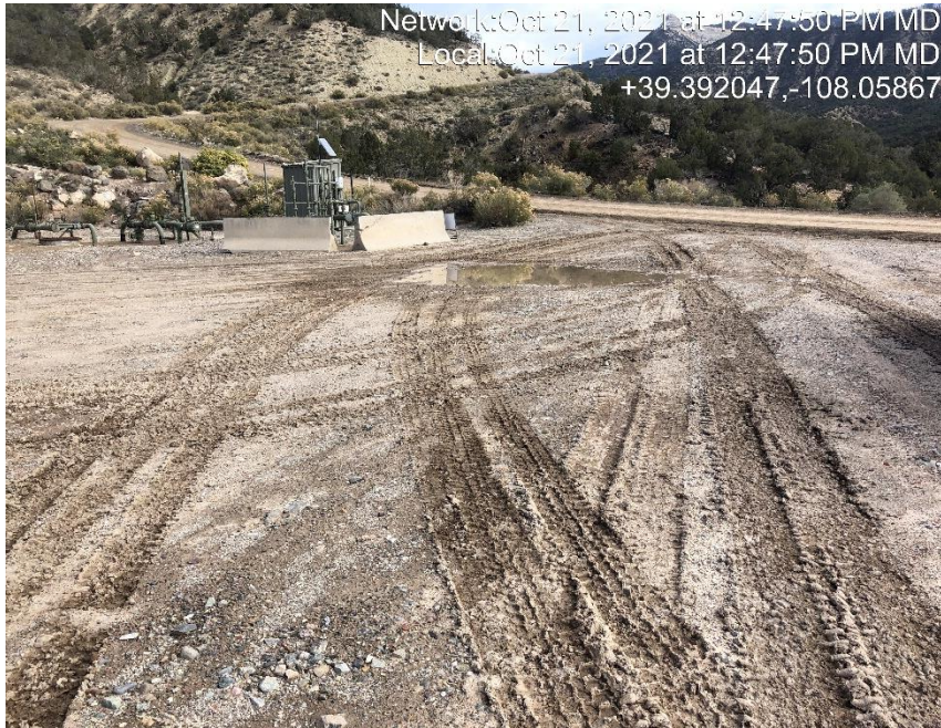
Photo #5130 No form of tracking BMP located at entrance to location.
