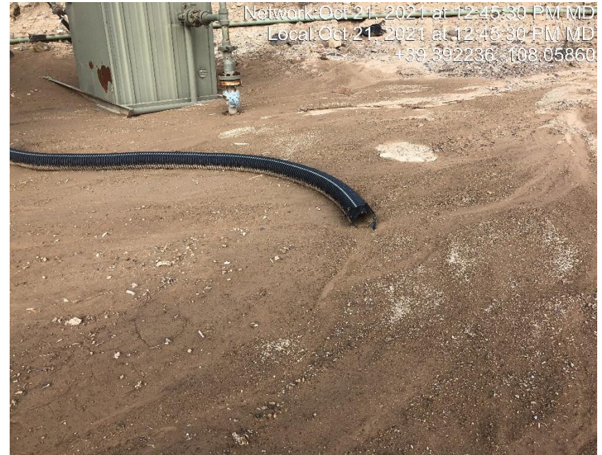
Photo #5126 Heating insulation open ended and not capped.
