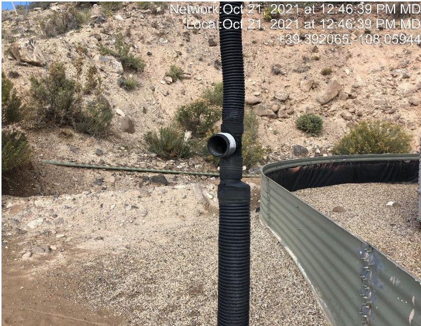
Photo #5127 Heating insulation open ended and not capped.
