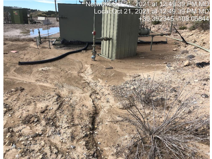
Photo #5132 Run on to location is not being controlled.
