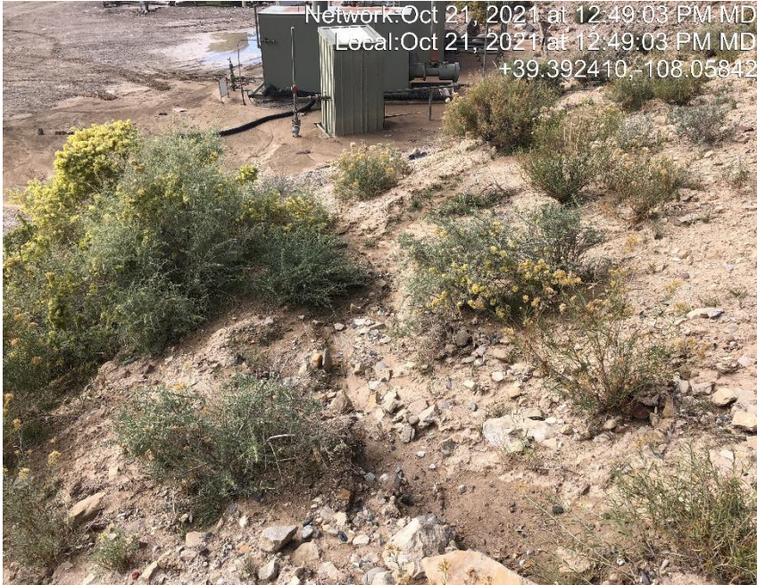
Photo #5131 Rill erosion occurring on cut slope.
