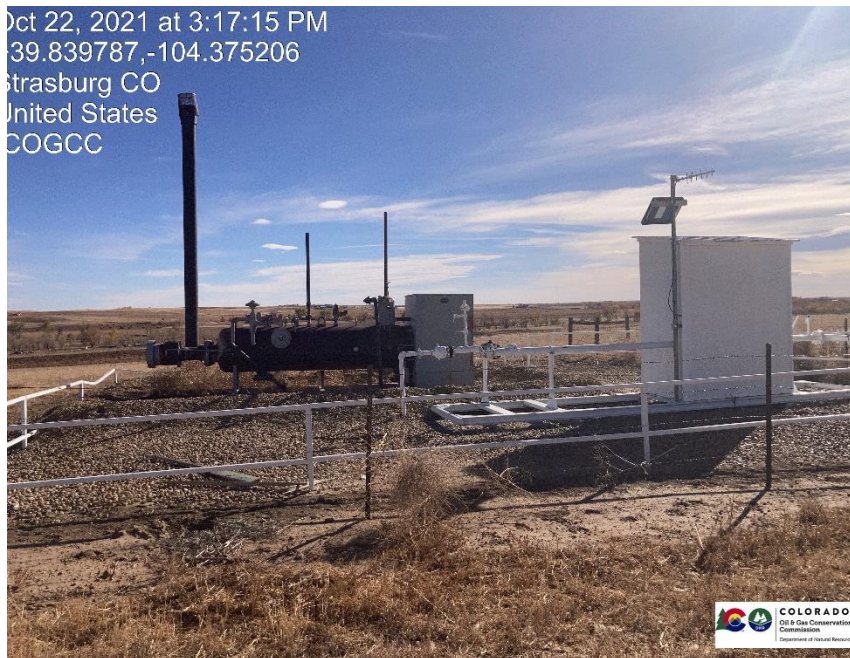
Pic 1 separator, gas meter run.
