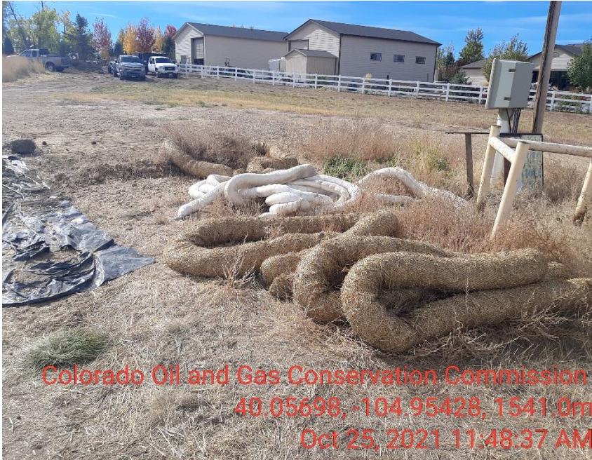
Photo 7 Waddles removed to haul off contaminated soil not staking material on site.
