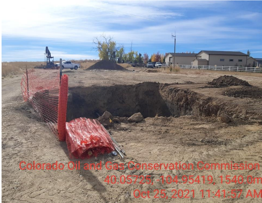
Photo 5 No location or excavation BMP's
