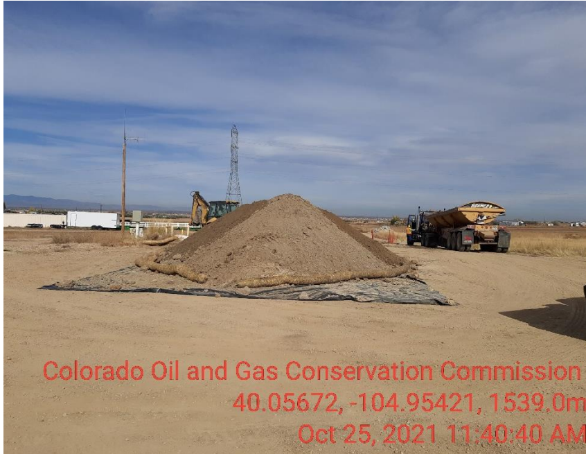
Photo 3 Straw waddles not properly installed.
