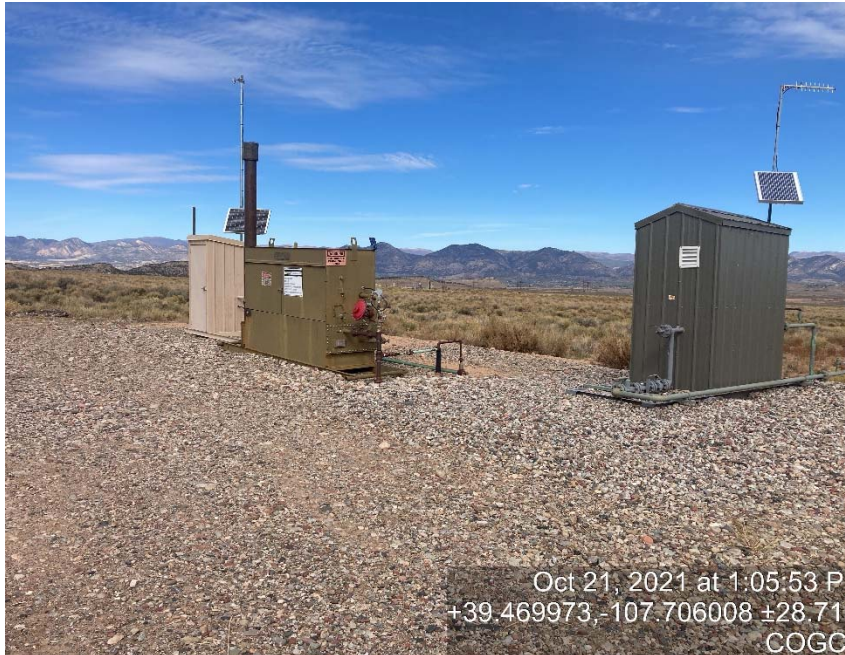
Location/Lack of labeling on glycol storage
