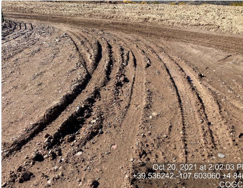
Lack of stabilization/compaction
