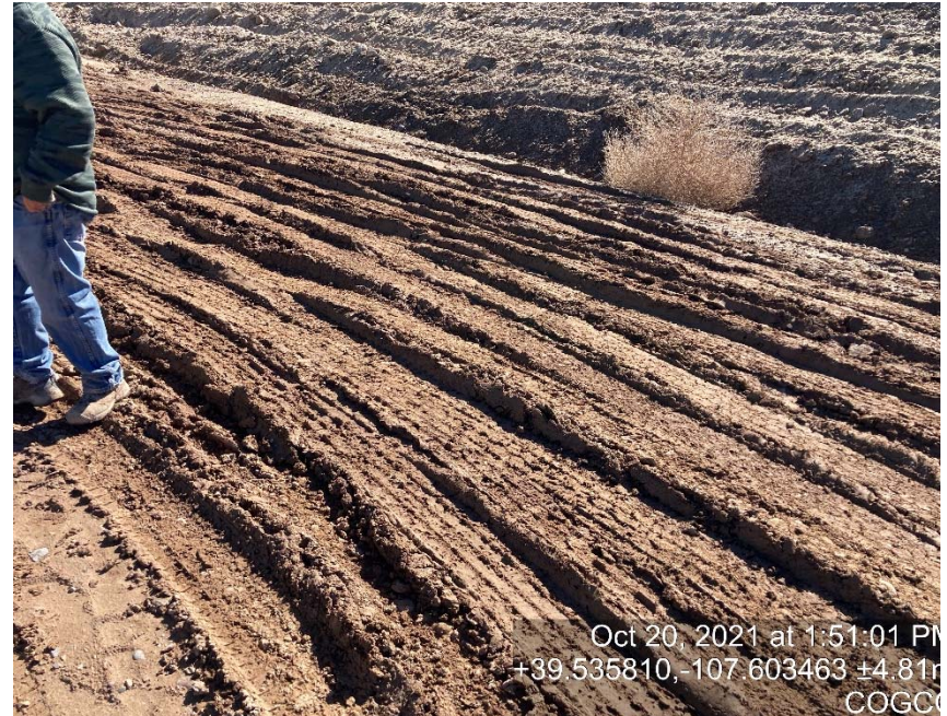
Lack of stabilization/compaction
