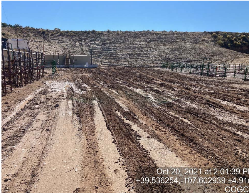
Lack of stabilization/compaction
