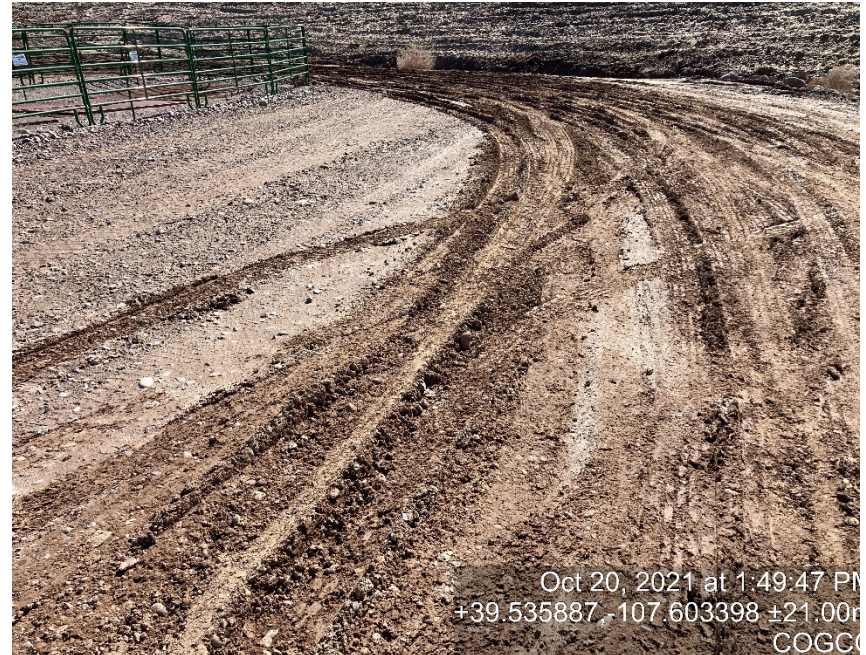
Lack of stabilization/compaction
