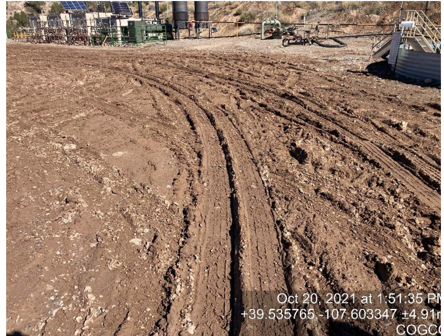
Lack of stabilization/compaction
