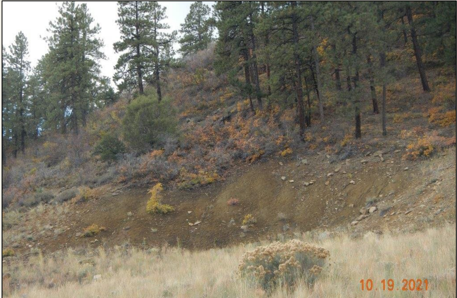
Photo 4. View of bare soils on the southern cut-slope, project area needs recontouring and stabilization.
