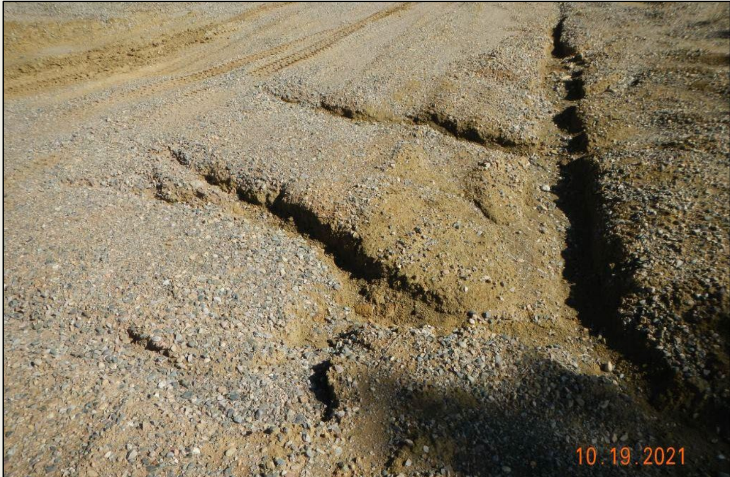
Photo 3. View of erosional rilling and channeling, approx. 1-2ft wide and deep at the well pad entrance, facing up-slope. This occurs where concentrated stormwater flows off of the well pad.
