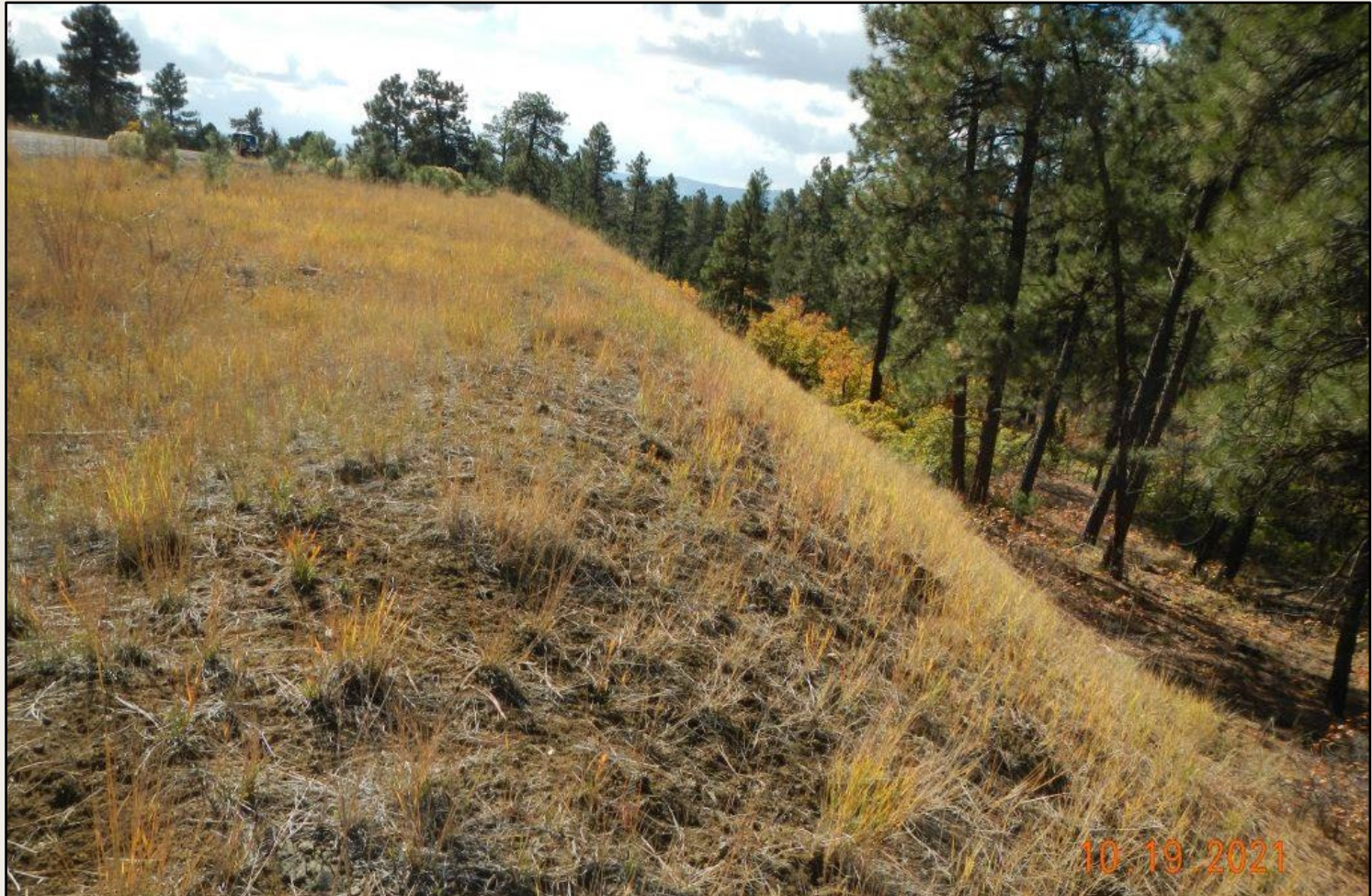
Photo 2. View of the western fill slope from the northwestern corner facing southward. Revegetation is progressing largely with western wheatgrass.
