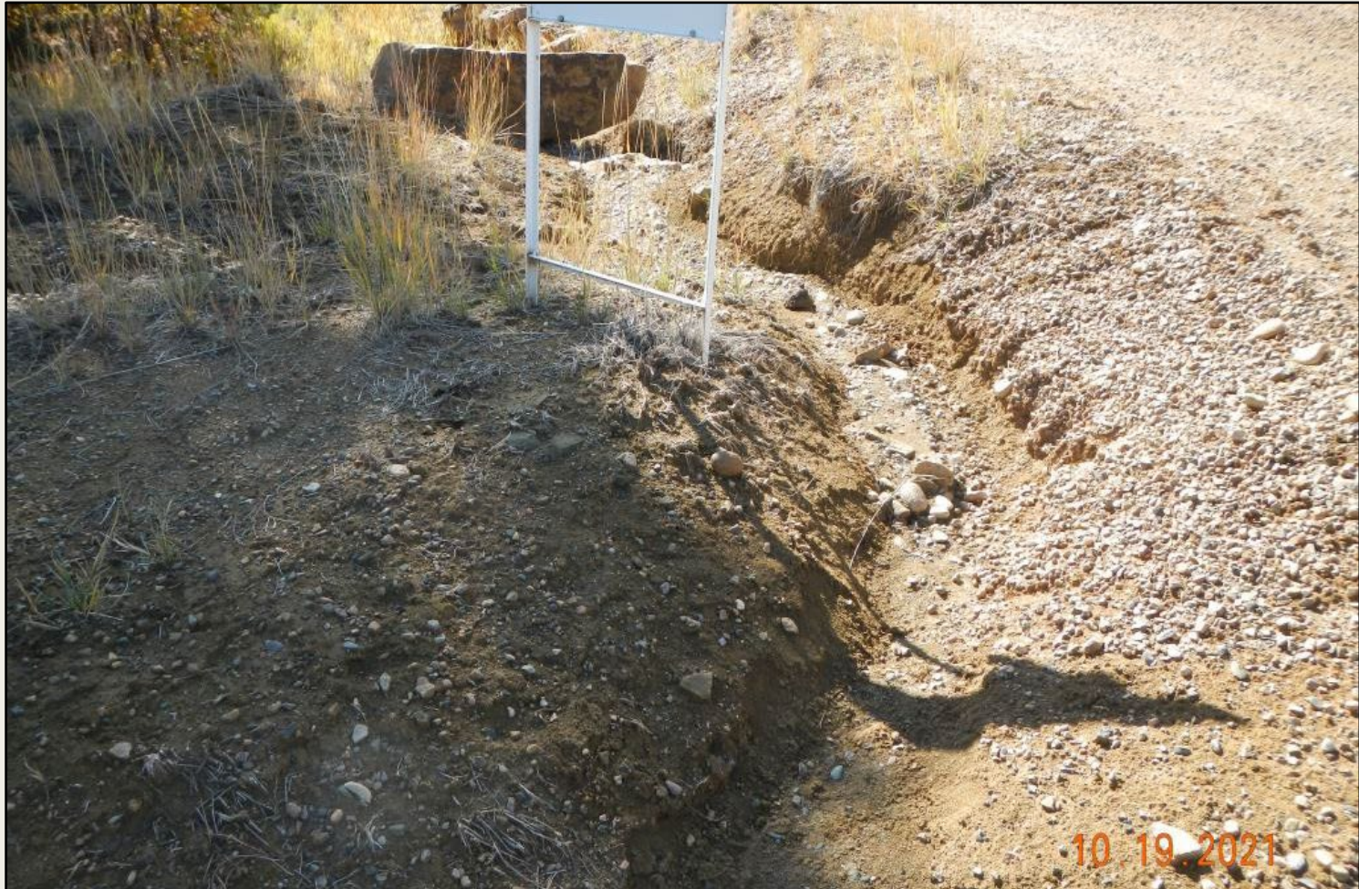
Photo 4. View of erosional channel, facing down-slope from photo 3, approx. 2ft wide and deep.
