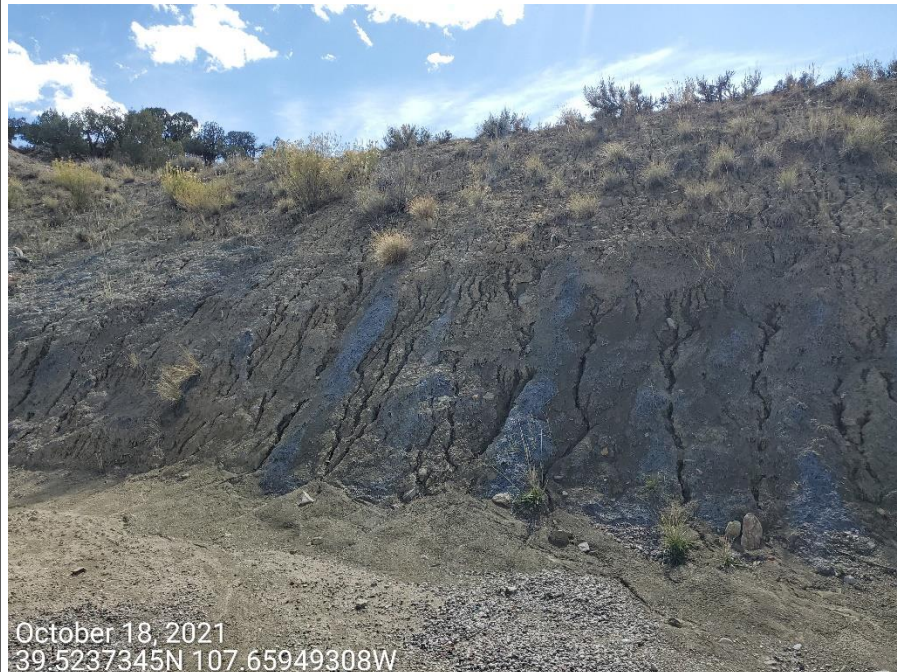
Photo 3: Photos taken from the cut slopes of the Location. Photos provide examples showing that control measures to protect and stabilize the slopes of the Location are missing or insufficient.
