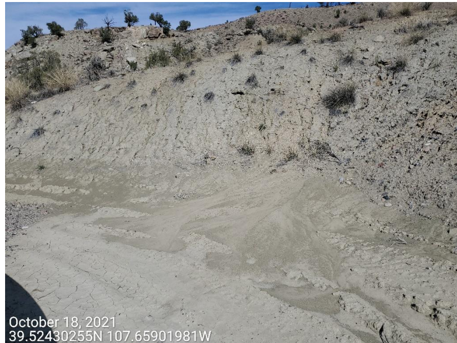
Photo 2: Photos taken from the cut slopes of the Location. Photos provide examples showing that control measures to protect and stabilize the slopes of the Location are missing or insufficient.
