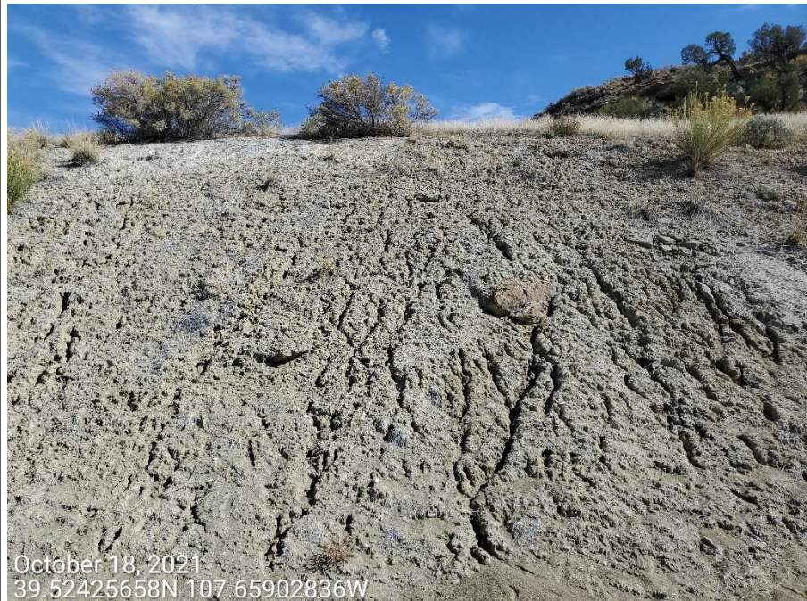
Photo 2: Photos taken from the cut slopes of the Location. Photos provide examples showing that control measures to protect and stabilize the slopes of the Location are missing or insufficient.
