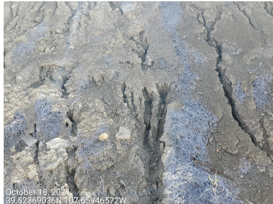
Photo 3: Photos taken from the cut slopes of the Location. Photos provide examples showing that control measures to protect and stabilize the slopes of the Location are missing or insufficient.
