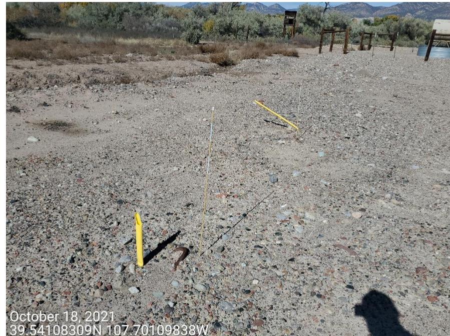
Photo 2: Photos show example of anchors on the location with markers that are missing, in disrepair, or not marked with an appropriate visible marker
