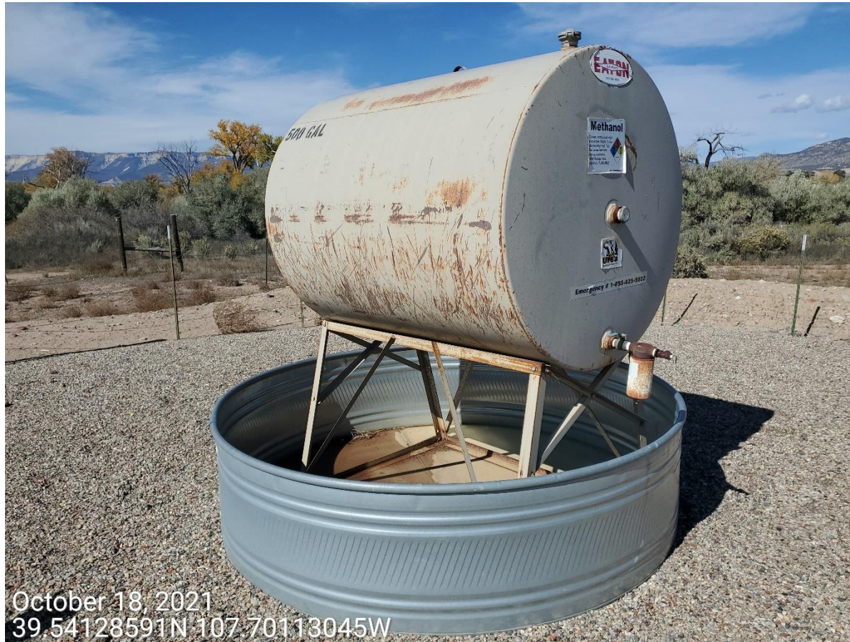
Photo 3: Photo shows protection devices to prevent wildlife access to the Methanol tanks containment BMP observed to be missing
