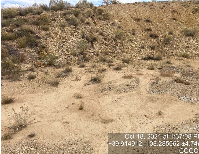
Lack of stabilization/erosion
