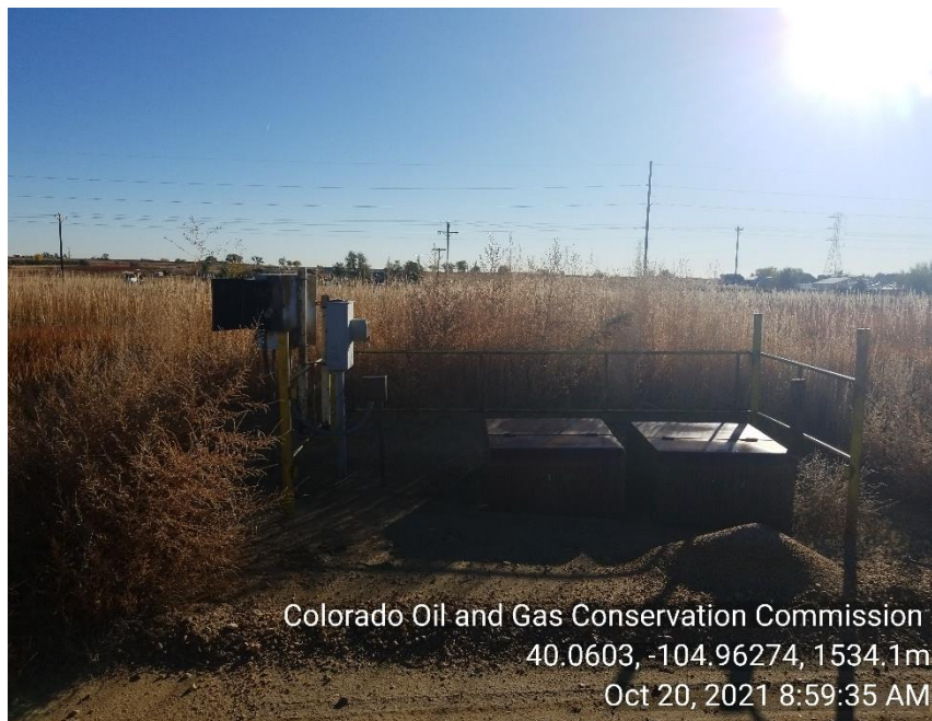
Photo 1 electric panel and breaker box open. Debris: dead weeds around electric equipment.
