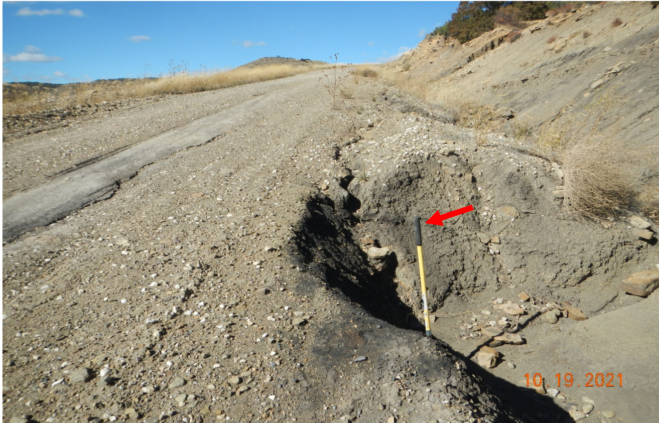
Photo 1. Facing west along the main road traveling to the well site. There is erosion along the road side. This area needs to be repaired and stabilized. Arrow points to 4.5 shovel placed in erosion channel. Previous corrective action was not performed.
