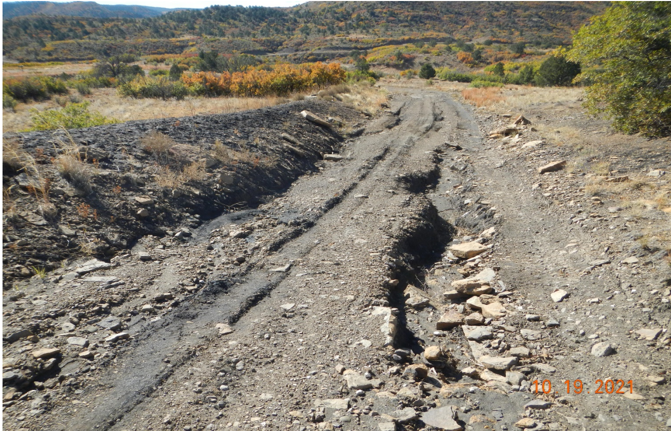
Photo 3. Facing south along the access road. There is erosion along the road that needs to be repaired and stabilized.
