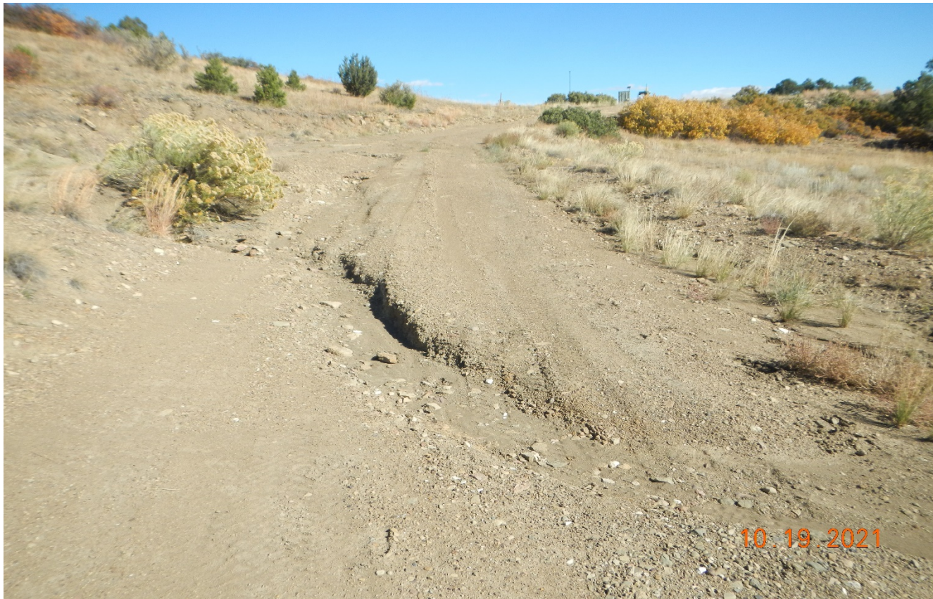
Photo 3. Facing northeast along the access road to the well site. There is an erosion channel across the access road.
