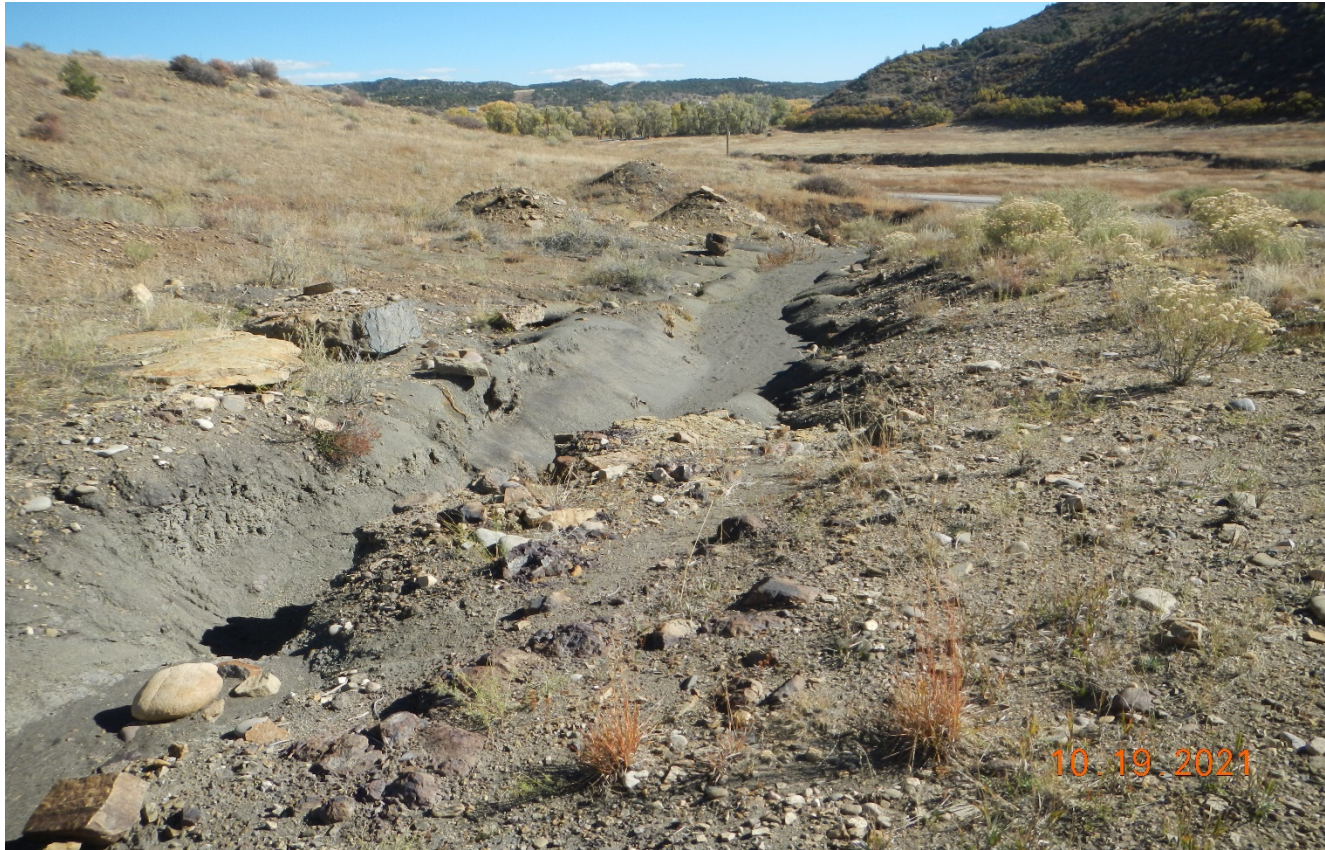
Photo 2. Facing back down from the previous photos shows the stormwater erosion which is directed toward the culvert and towards the main Lorencito road.
