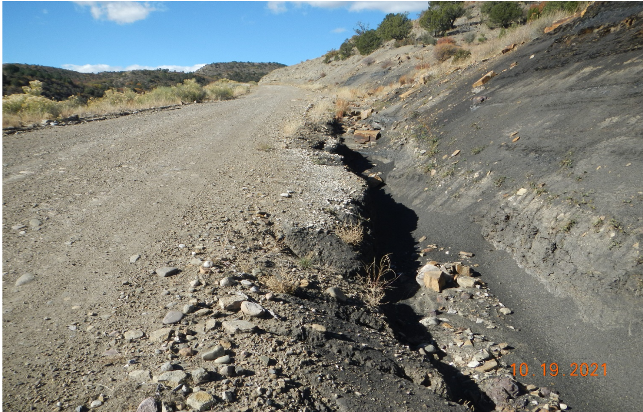
Photo 1. Facing southwest along the main road to the well site. There is erosion along the road which is causing sediment accumulation at the culvert and at the main road in Lorencito Canyon. Previous corrective action was not performed.
